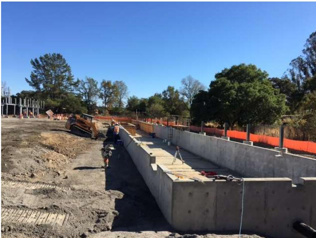
Figure 4 – Backfilling and compacting fill along east side of SPCC pond – view south, October 5, 2017.
