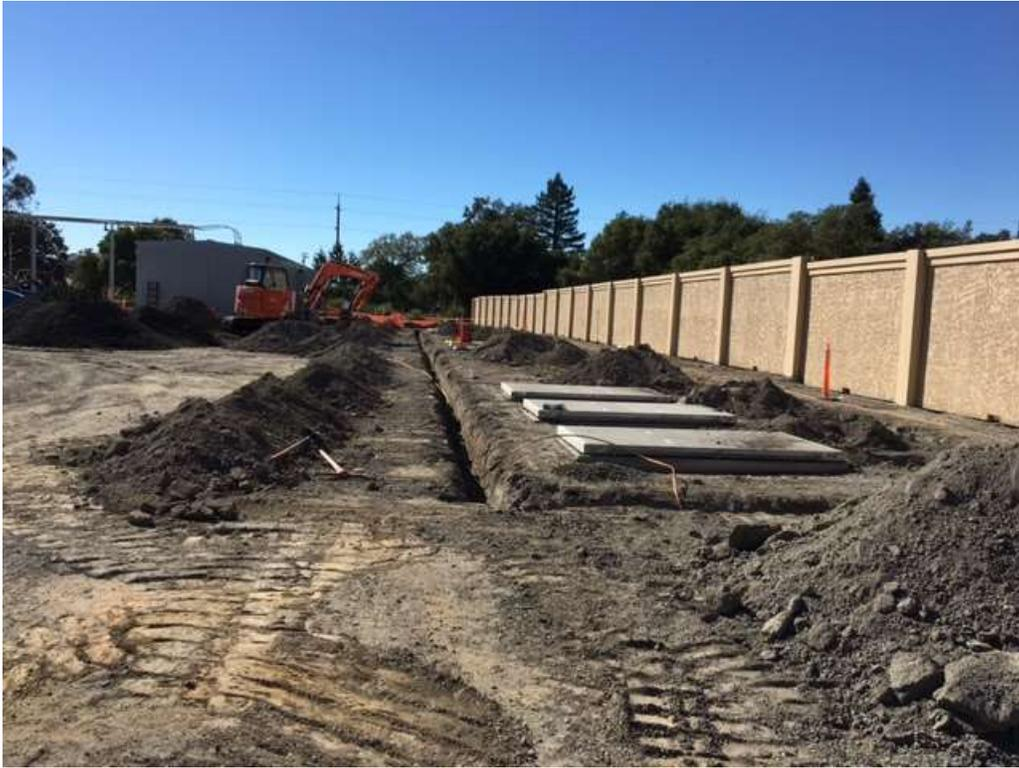
Figure 1 – Conduit trenching on north side of switchgear building – view west, October 27, 2017.
