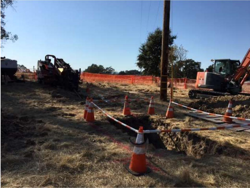
Figure 1 – HDD entrance pit and equipment set-up – view west-northwest, October 31, 2017.
