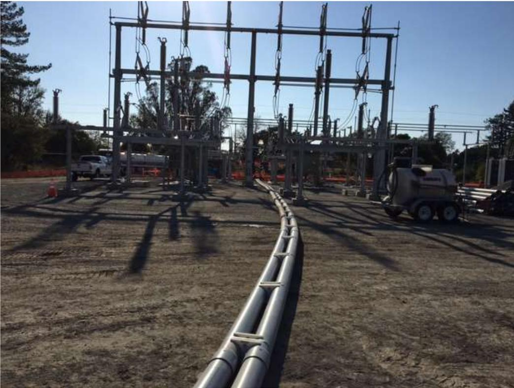
Figure 4 – Conduit ready to be pulled through HDD bore – view west, October 31, 2017.
