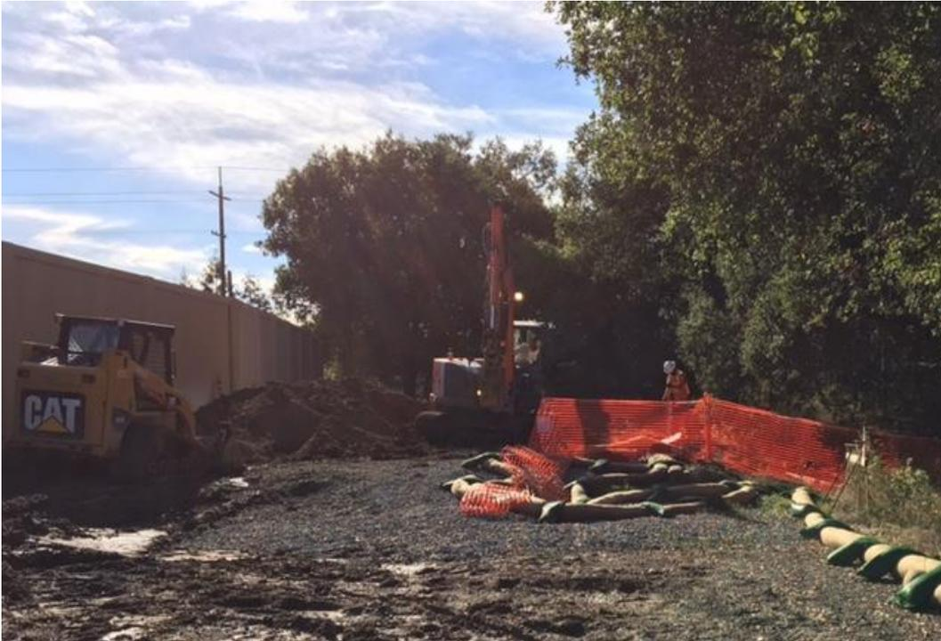
Figure 1 – Excavating trench for drainage pipe in northwest corner of substation site – view west, November 14, 2017.
