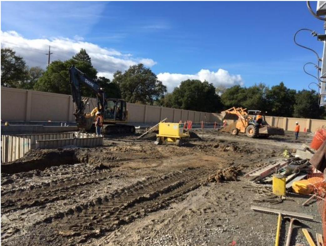
Figure 2 – Pull box and conduit trenching on east side of SPCC pond – view northwest, November 14, 2017.
