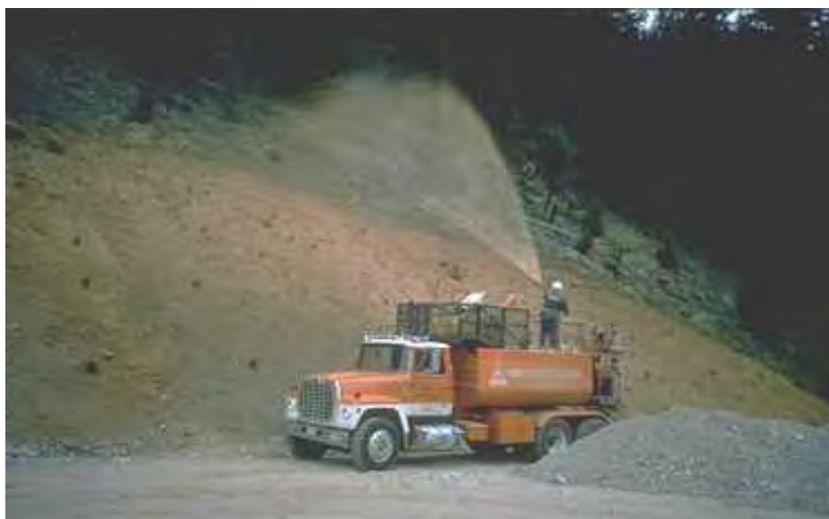
Applying hydraulic mulch.
