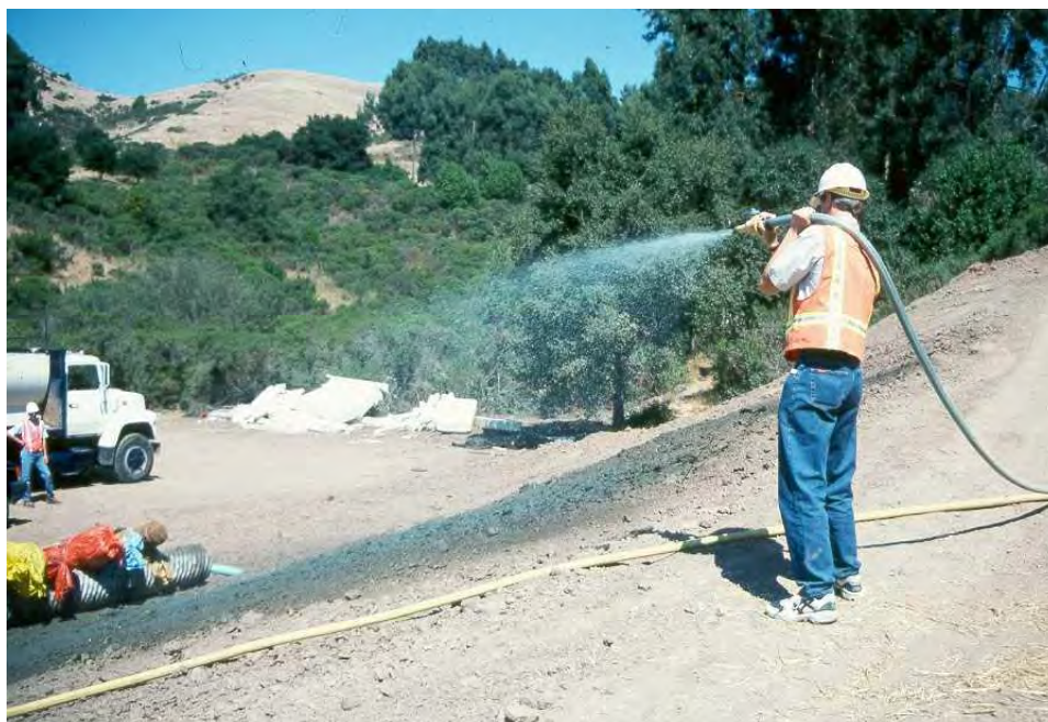
Applying hydroseed.
