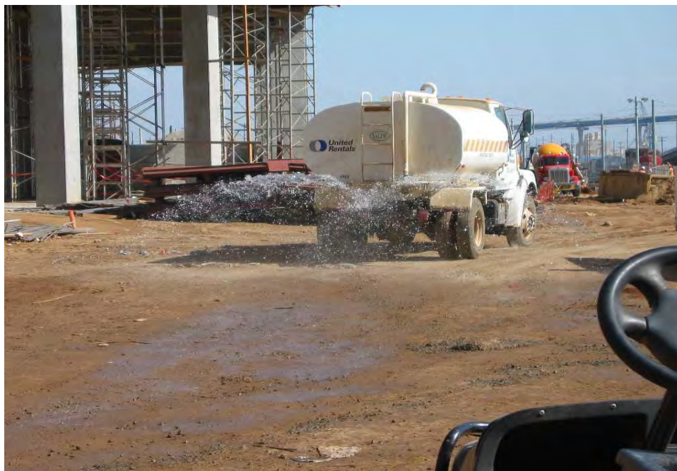
Water being applied for dust control.
