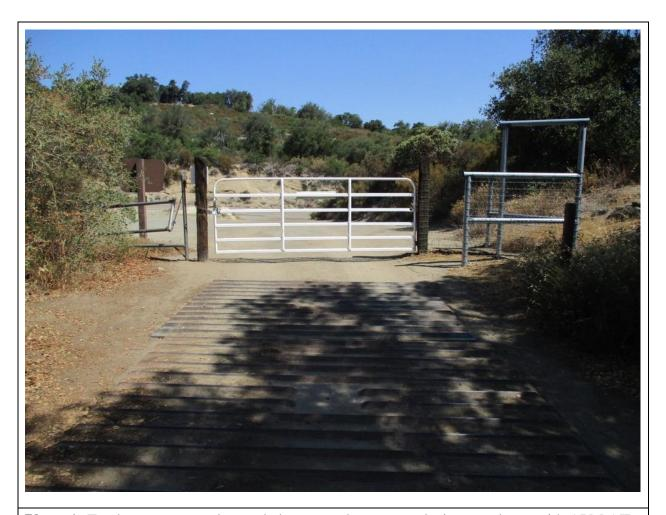
**Photo 1:** Track-out was not observed along paved access roads, in accordance with APM AIR-05 and the SWPPP (APM HYD-09, MM HYD-1, MM BIO-7). Rattle plates were documented at the ingress/egress of Love Valley Road, and the gate was kept closed and locked to prevent unauthorized access in accordance with MM REC-2.
