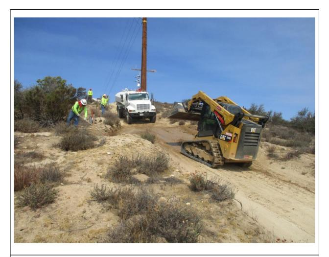
**Photo 2:** During water bar grading and energy dissipater maintenance between Poles Z44282 and Z44281 (TL 6931), a 150-gallon water truck was used to aid in soil compaction and dust control in accordance with APM AIR-02 and to comply with the CFPPP fire prevention matrix (off CNF land - FPI elevated) (MM FF-1)
