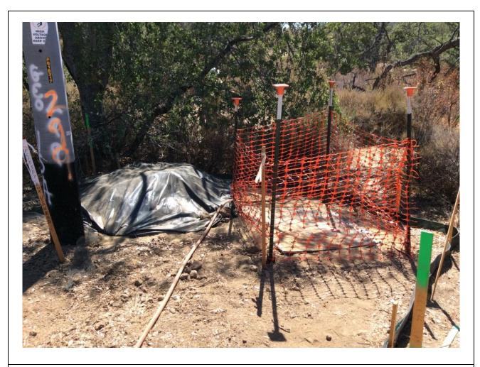
**Photo 4:** A completed pole hole at Pole P618317 (TL682) was observed securely covered to prevent wildlife entrapment in accordance with MM BIO-23. In addition, the spoils stockpile was covered with plastic sheeting to prevent erosion in accordance with the Erosion Control Plan and SWPPP (APM HYD-09, MM HYD-1, MM BIO-7).
