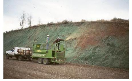
Applying a tackifier using a trailer mounted pump and hose.
