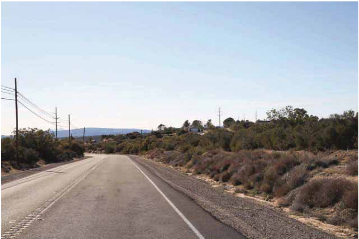
4. SR-94 looking west *
