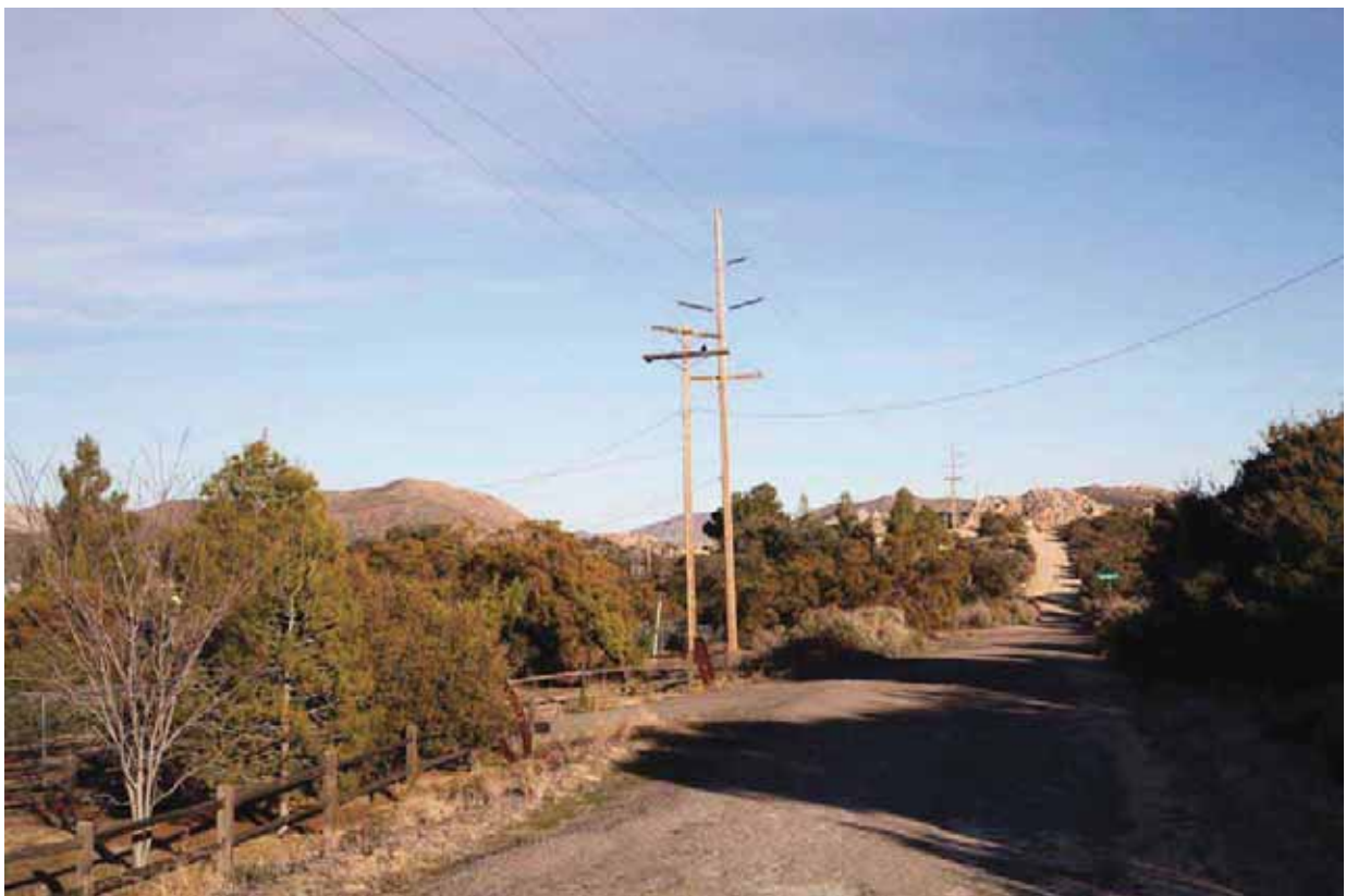
8. Ross Avenue at McCain Lane looking east
