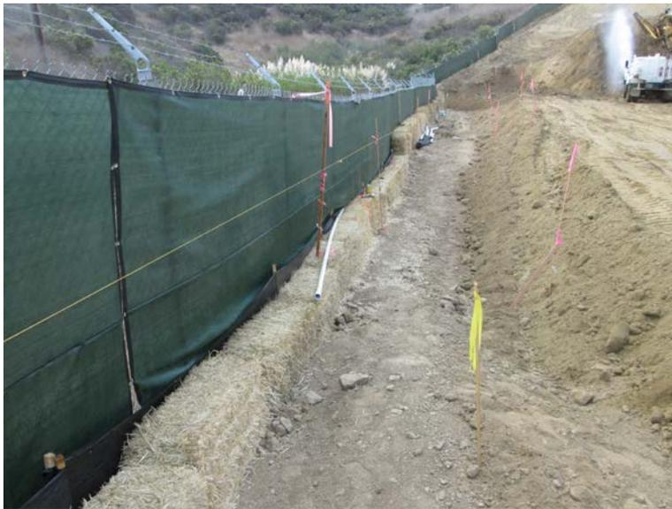
**Photo 4:** In accordance with APM-HYD-1, storm water control BMPs were used along the eastern site perimeter to prevent erosion and silt laden runoff from entering the adjacent wetland ESA.
