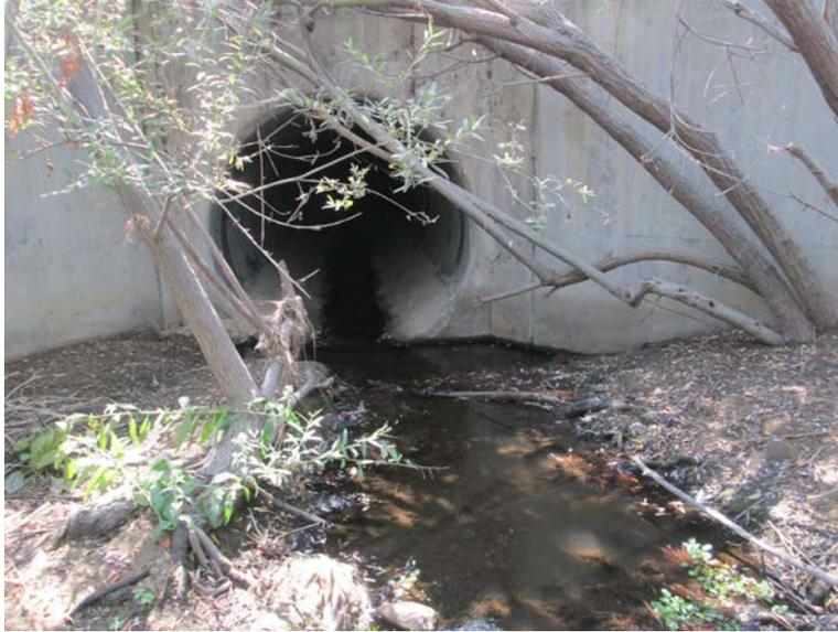
**Photo 3:** Groundwater dewatering discharge piping was removed from the culvert and surrounding wetland habitat located to the east of the eastern site perimeter. A biological monitor was present during the removal of the discharge piping.
