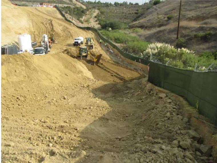
**Photo 1:** Earthwork activities occurring along the eastern limits of the project site following the completion of groundwater removal activities.
