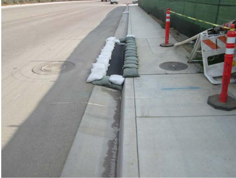
**Photo 5:** In accordance with APM-HYD-1, inlet protection BMPs were utilized at all applicable storm drains to minimize the potential for sediment laden water from entering waterways.
