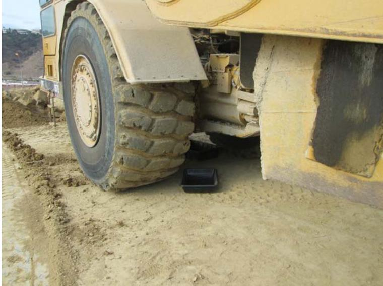
**Photo 6:** In accordance with APM-HYD-1, secondary containment was used under staged construction equipment to prevent potential leaks from being discharged into the soil.
