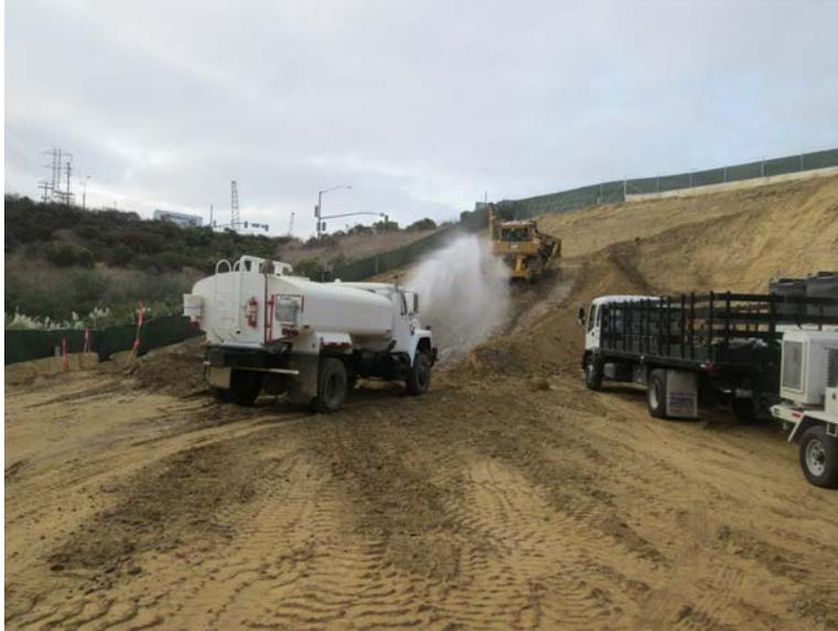
**Photo 7:** In accordance with APM-HYD-1, water was applied in areas of active construction and along access roads to prevent wind erosion and dust.
