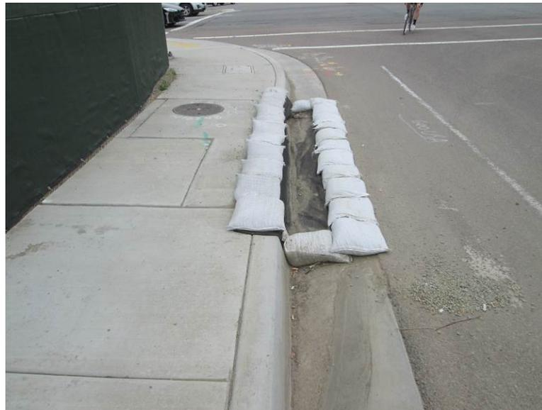
**Photo 2:** In accordance with APM-HYD-1, inlet protection BMPs are being utilized at storm drains to minimize the potential for sediment laden water from entering waterways.
