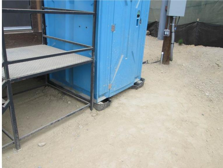
**Photo 3:** In accordance with APM-HYD-1, secondary containment has been placed beneath portable bathrooms to prevent potential leaks from being discharged into the soil.
