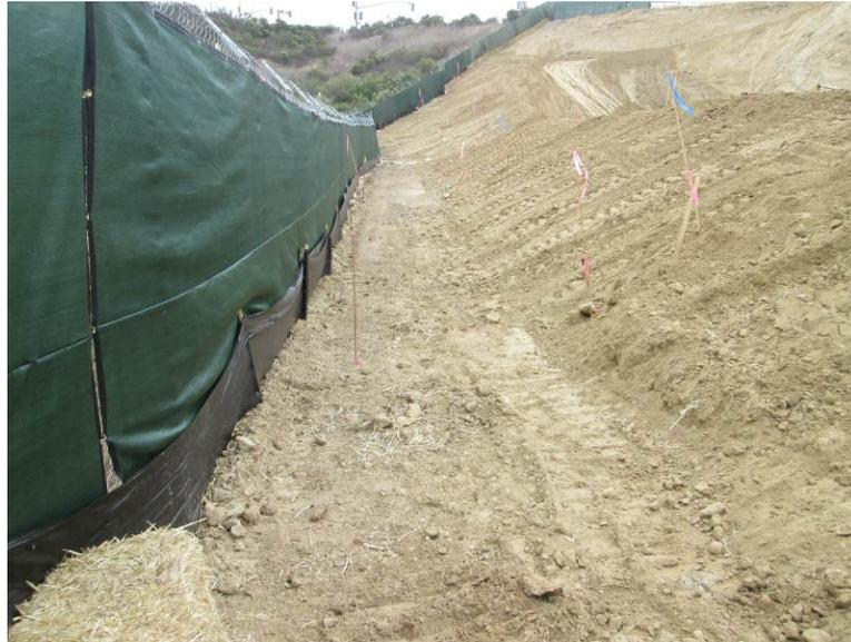
**Photo 1:** In accordance with APM-HYD-1, BMPs consisting of silt fence have been installed along the eastern perimeter of the project site.
