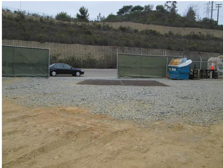
**Photo 6:** In accordance with APM-HYD-1, rumble plates and a rock apron have been installed at the project entrance to minimize the potential for sediment being tracked onto Mira Sorrento Place.
