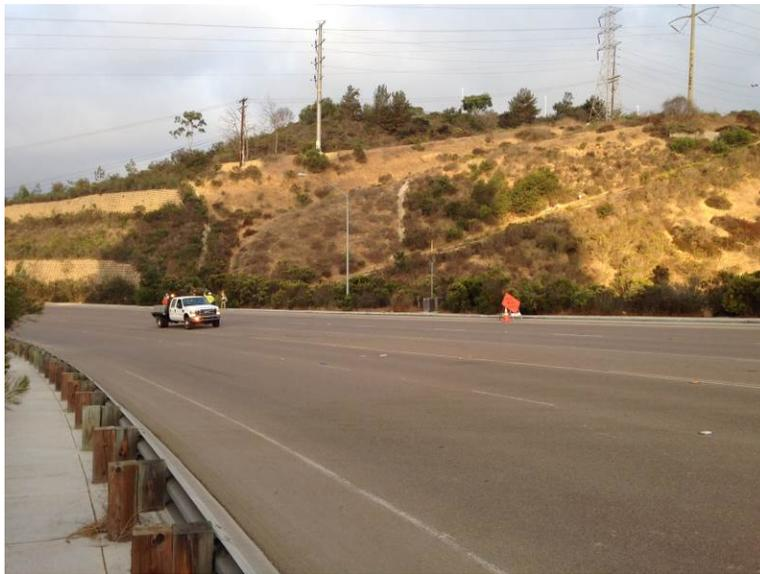
**Photo 4:** In accordance with MM-TT-1, traffic control signage is placed along Mira Sorrento Parkway notifying motorists of construction activities.
