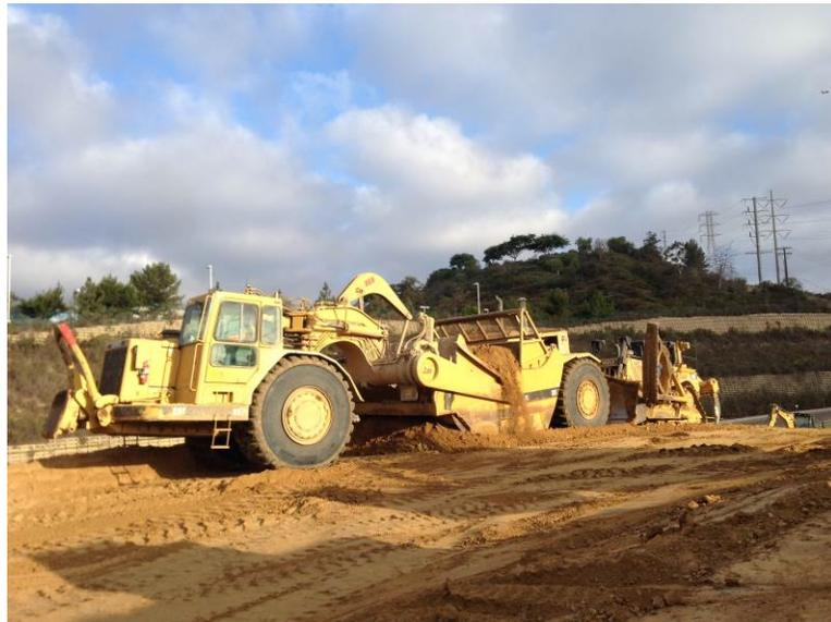
**Photo 2:** Earthwork activities along the northern project limits were completed during this reporting period to establish an access route for importing fill material that will be utilized for erecting the retaining wall.
