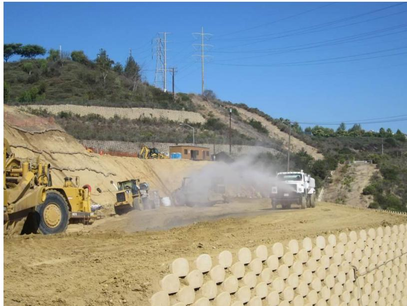
**Photo 2:** Construction crews utilize water for dust control and compaction purposes.
