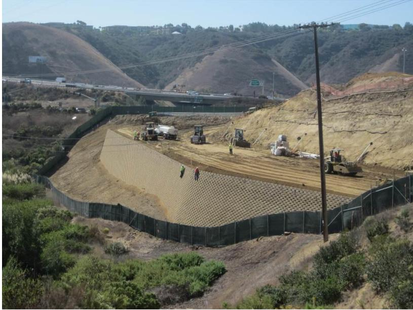
**Photo 1:** Construction activities associated with erecting the eastern retaining wall continued during this reporting period.
