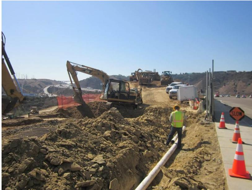
**Photo 3:** Storm drain piping being installed along the southern limits of Mira Sorrento Place.
