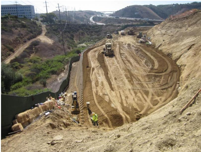
**Photo 4:** Silt fence and straw bales are being maintained along the eastern limits of the project site in accordance with the SWPPP.
