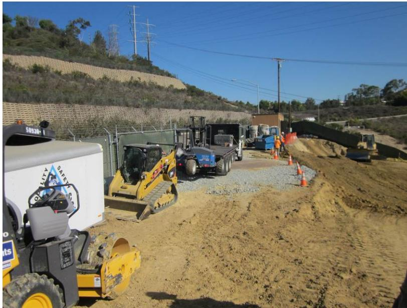
**Photo 4:** A rock apron and rattle plate is being maintained at the project entrance to minimize the potential for trac-out along Mira Sorrento Place.
