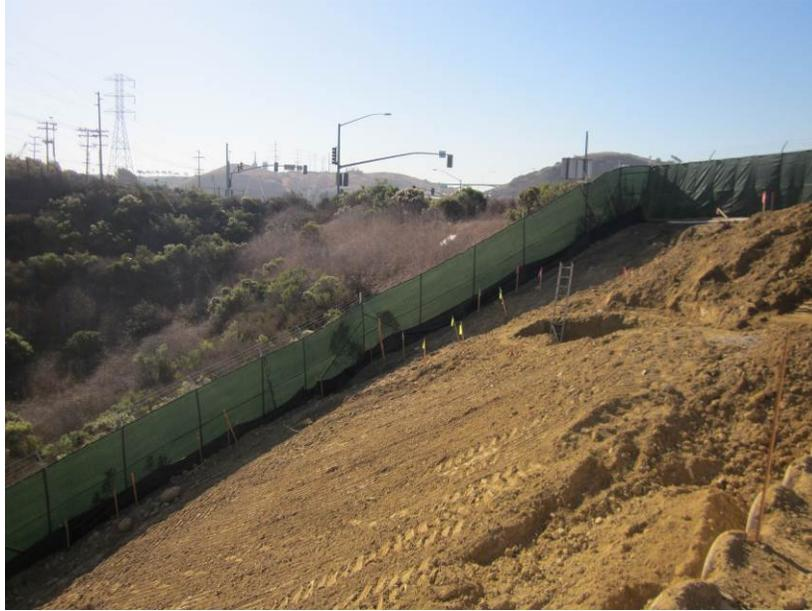
**Photo 3:** In accordance with MM-HYD-1, Best Management Practices (BMPs) consisting of silt fence and straw bales are being maintained along the eastern perimeter of the project site.
