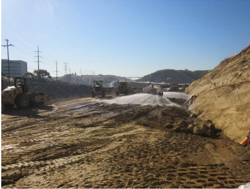
**Photo 1:** Soils being compacted through use of heavy construction equipment and water along the top of the retaining wall.
