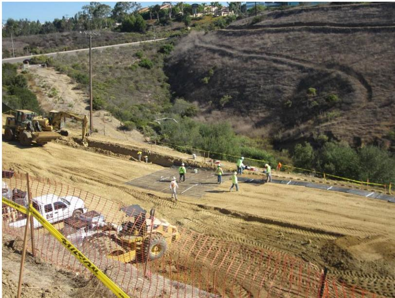
**Photo 2:** Geogrid fabric is placed between each layer of retaining wall blocks in accordance with the engineering specifications.
