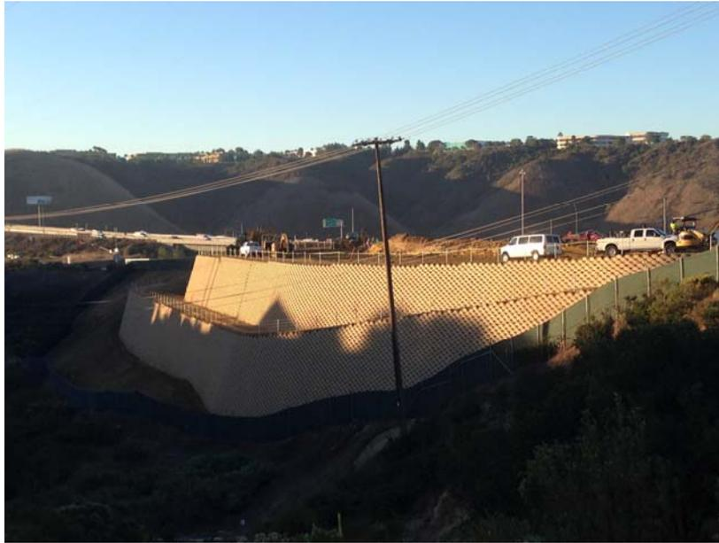
**Photo 1:** Construction crews have completed constructing both retaining walls. Safety fencing was observed being installed along the perimeter of the retaining walls.
