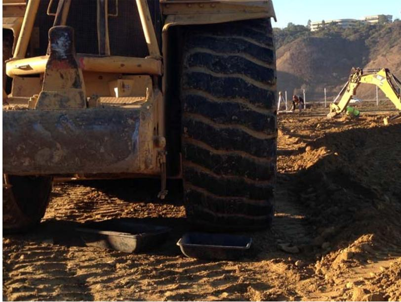
**Photo 3:** In accordance with MM-HYD-1, containment bins are placed beneath construction equipment.
