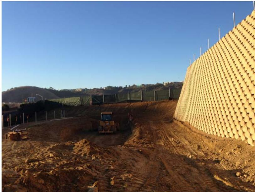
**Photo 2:** Excavation associated with constructing the retention basin located in the southwest corner of the project site continued during this reporting period.
