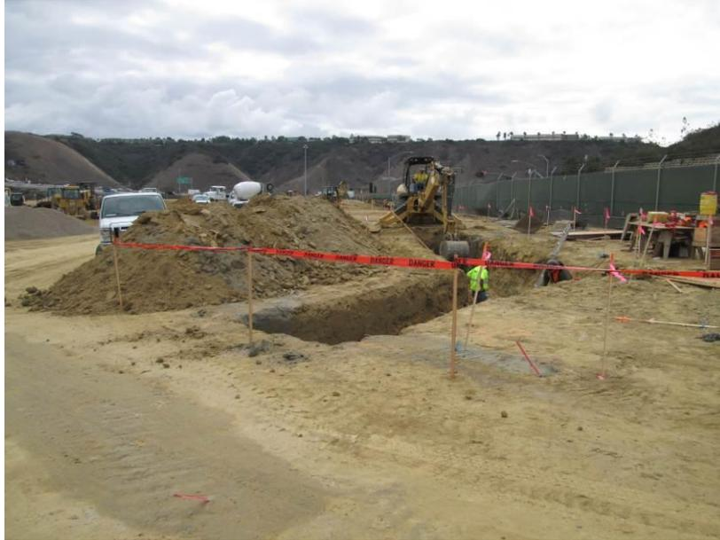
**Photo 1:** Construction continued on the foundation for the perimeter screening wall during this reporting period. The screening wall is being constructed to minimize visual contrast with surrounding areas in accordance with APM-AES-2.
