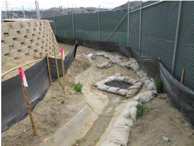
**Photo 3:** In accordance with APM-HYD-1, inlet protection BMP's were being utilized at storm drains located along the project site perimeter and were observed to be maintained in good working order.
