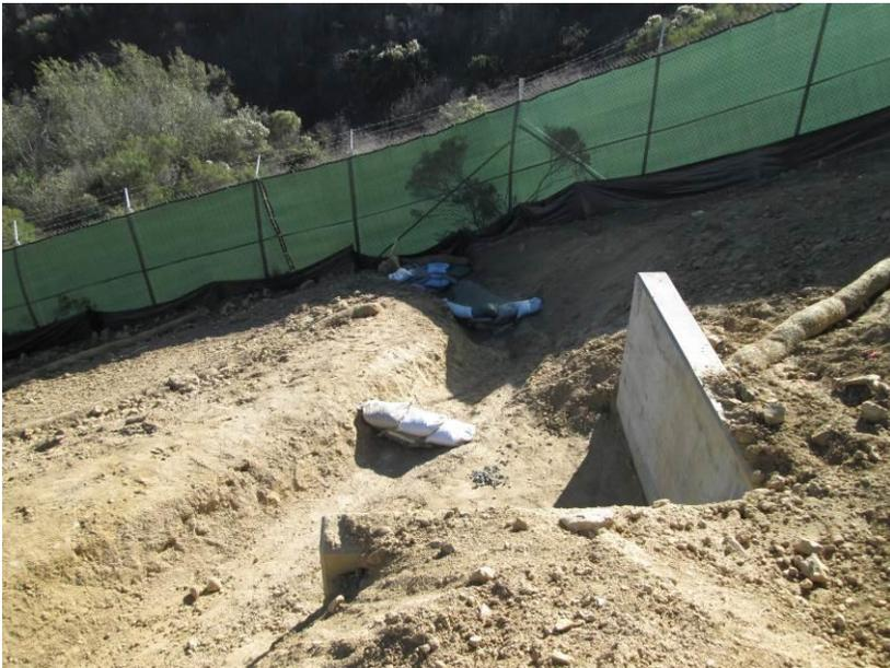
**Photo 2:** In accordance with APM-HYD-1, gravel bag check dams were observed in a drainage canal, and straw wattles, silt fencing, and gravel bags were observed where the canal meets the project site perimeter.
