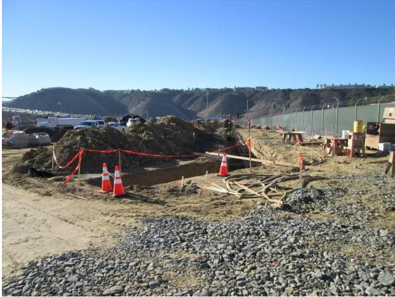
**Photo 1:** Construction crews continued work associated with the foundation for the perimeter screening wall during this reporting period.
