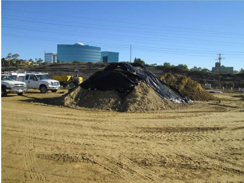
**Photo 3:** Dirt stockpiles were watered and/or covered to minimize or prevent wind erosion and dust creation in accordance with APM-HYD-1
