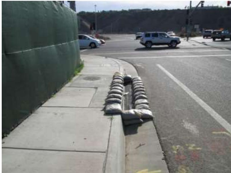
**Photo 4:** Gravel bags and filter fabric were observed being maintained at stormwater inlet structures located adjacent to construction activities in accordance with APM-HYD-1
