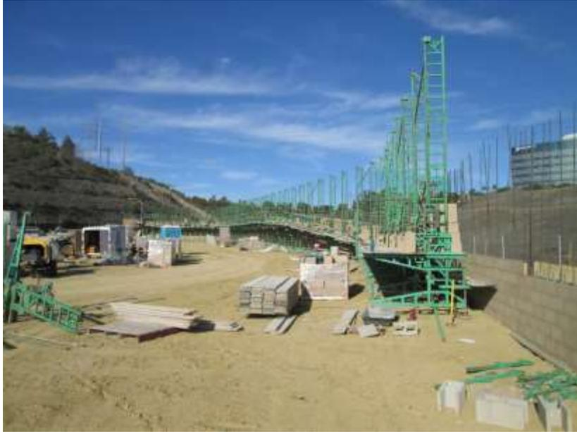
**Photo 1:** Construction crews continued work associated with erecting the screening wall along the perimeter of the substation pad.
