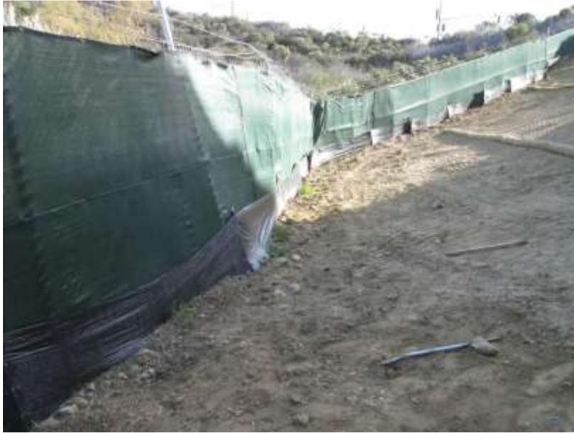
**Photo 3:** Silt fencing was observed being maintained along the eastern limits of the substation adjacent to environmental sensitive areas in accordance with APM-HYD-1
