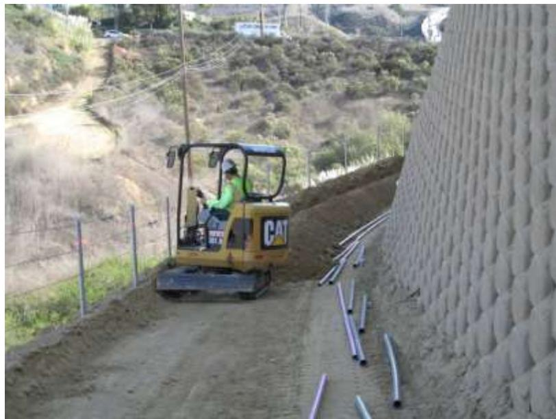
**Photo 2:** Crews were observed placing conduit and irrigation pipes between the Tier 1 and Tier 2 retaining walls.
