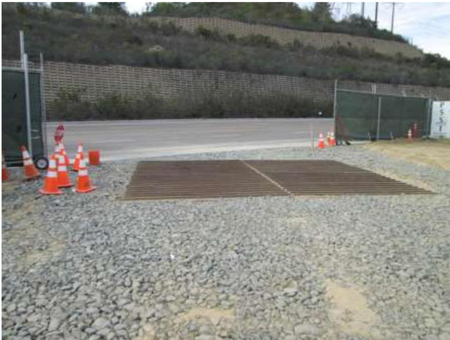
**Photo 4:** A rock apron and rattle plate were observed being maintained at the construction site entrance to minimize trac-out in accordance with APM-HYD-1.
