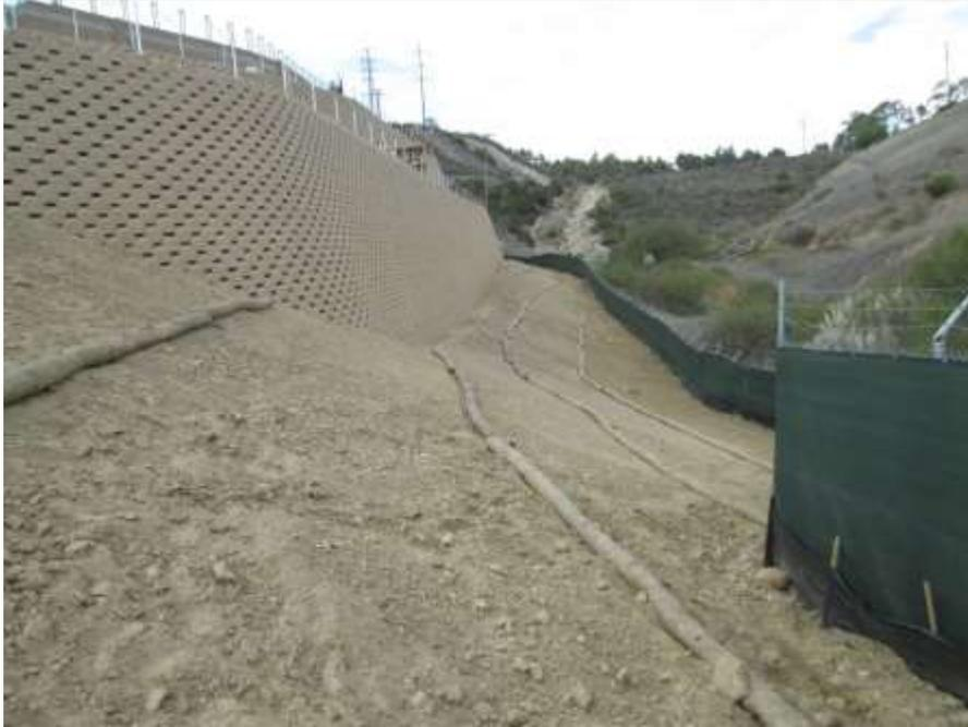
**Photo 3:** Silt fencing and straw wattles were observed being maintained along the eastern limits of the substation adjacent to environmental sensitive areas in accordance with APM-HYD-1
