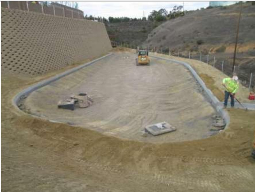
**Photo 2:** Crews were observed completing fine grading for the drainage basin located in the southwest portion of the project site.
