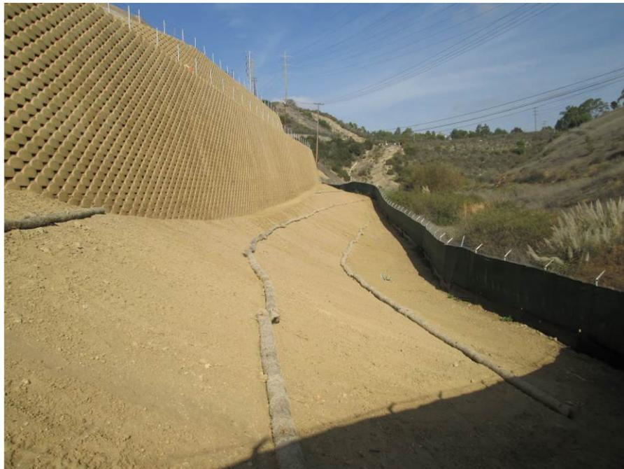
**Photo 4:** BMP's consisting of straw wattles and silt fence are being maintained along the eastern slopes of the project site in accordance with the SWPPP and APM-HYD-1.
