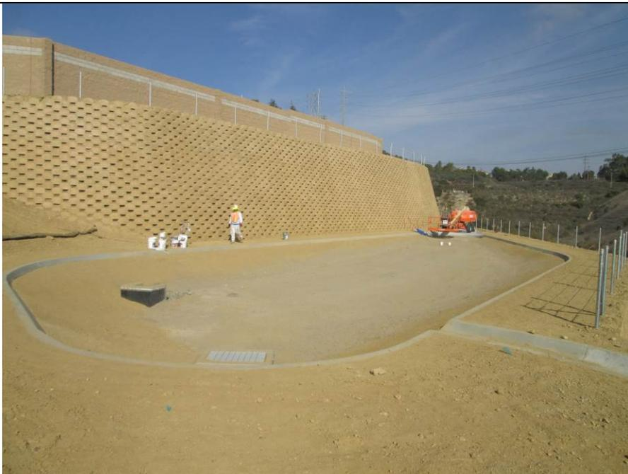
**Photo 2:** Construction crews were observed completing construction activities associated with finalizing the drainage basin located in the southwest portion of the project site.
