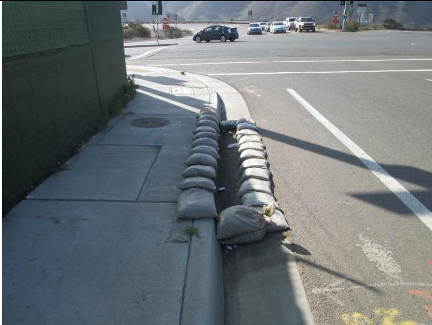
**Photo 3:** Gravel bags and filter fabric are being maintained at storm drains inlet structures located adjacent to the project site in accordance with the SWPPP and APM-HYD-1.
