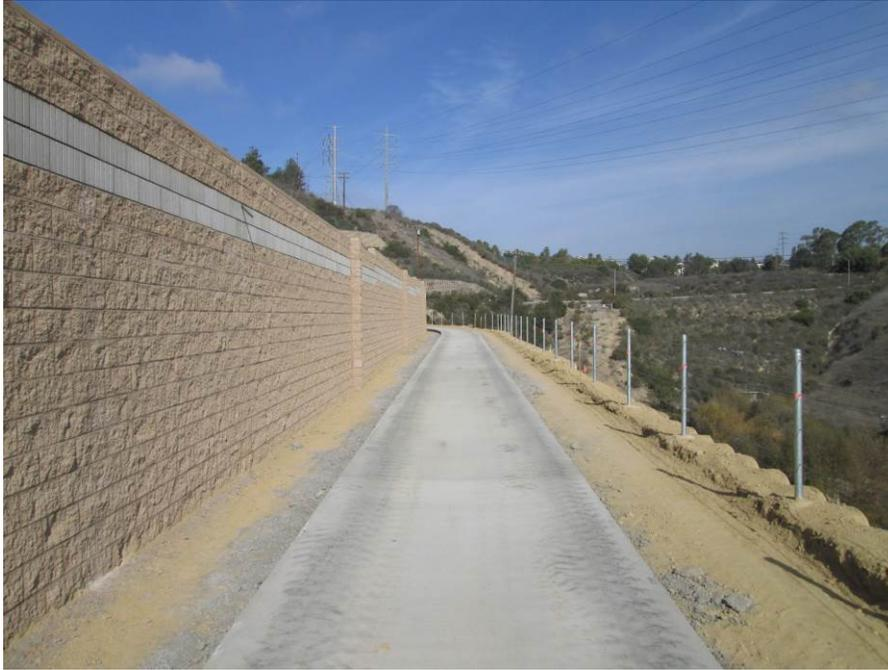
**Photo 1:** Construction crews were observed constructing an access road adjacent to the screening wall in order to provide access for maintenance activities at the drainage basin.
