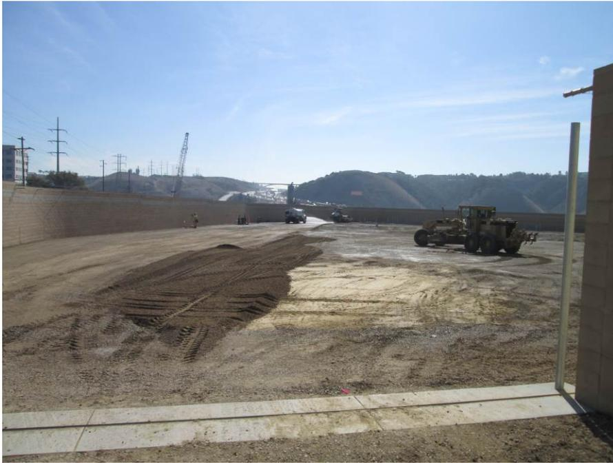
**Photo 1:** Construction crews were observed placing class 2 fill at the substation pad.
