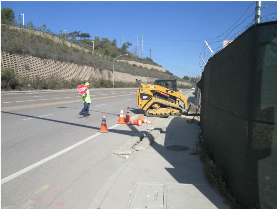
**Photo 4:** A flagger was observed being utilized when construction equipment had to temporarily access Mira Sorrento Place in accordance with the traffic control plan and MM-TT-1.
