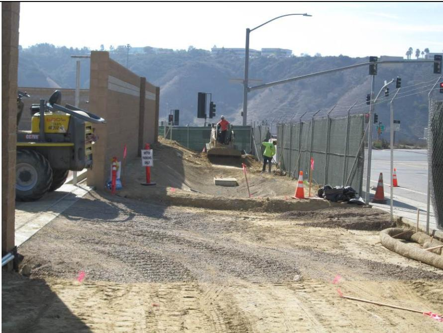
**Photo 2:** Construction crews were observed grading along the perimeter of the screening wall in preparation for the import of topsoil to be utilized for landscaping.
