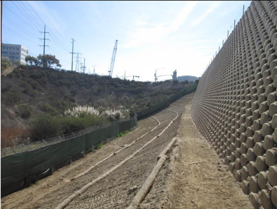
**Photo 3:** Silt fencing and straw wattles are being maintained along the eastern perimeter in accordance with the project SWPPP and APM-HYD-1.
