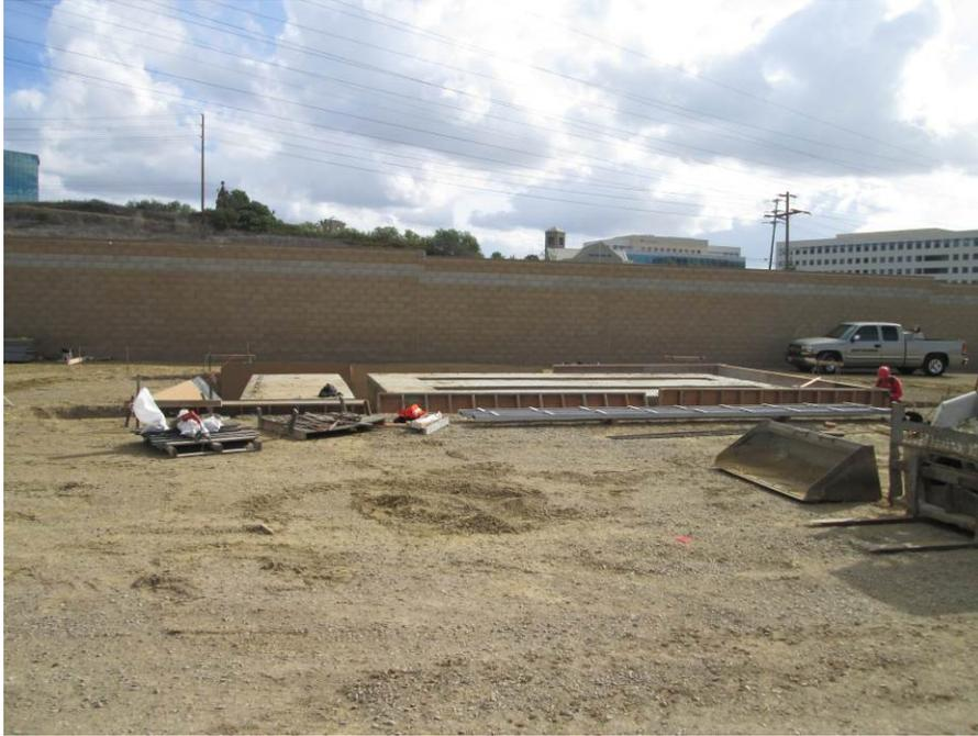
**Photo 1:** Construction crews were observed building foundations for the transformer pads during this reporting period.
