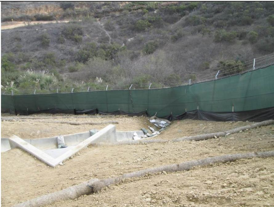
**Photo 2:** Silt fencing, straw wattles, and gravel bag check dams are being maintained along the eastern perimeter of the project site in accordance with the project SWPPP and APM-HYD-1.
