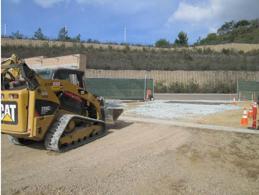
**Photo 3:** Construction crews were observed installing additional rocks to maintain the rock apron to minimize the potential for trac-out along Mira Sorrento Place in accordance with the project SWPPP and APM-HYD-1.
