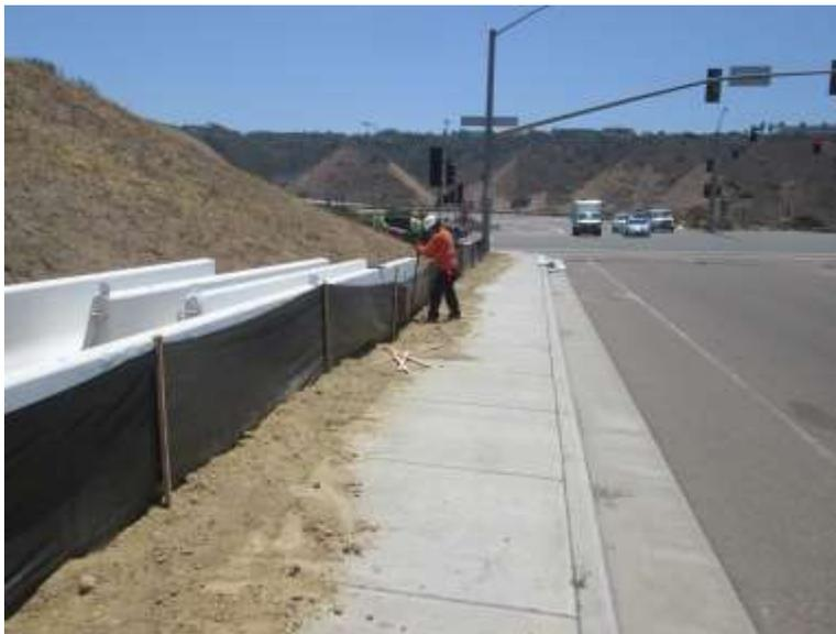
**Photo 2:** BMP's consisting of silt fence were installed along the perimeter of the project site in accordance with the SWPPP and MM-HYD-1.
