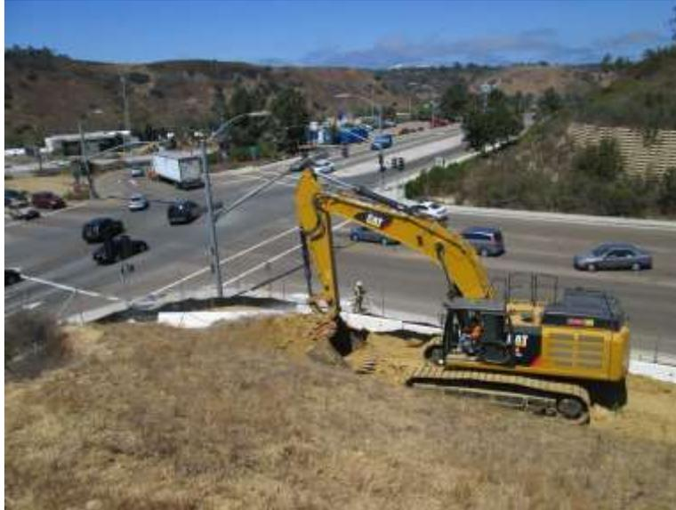
**Photo 1:** Construction crews completing ground disturbance activities within the approved work limits to establish an access road along the perimeter of the project site.
