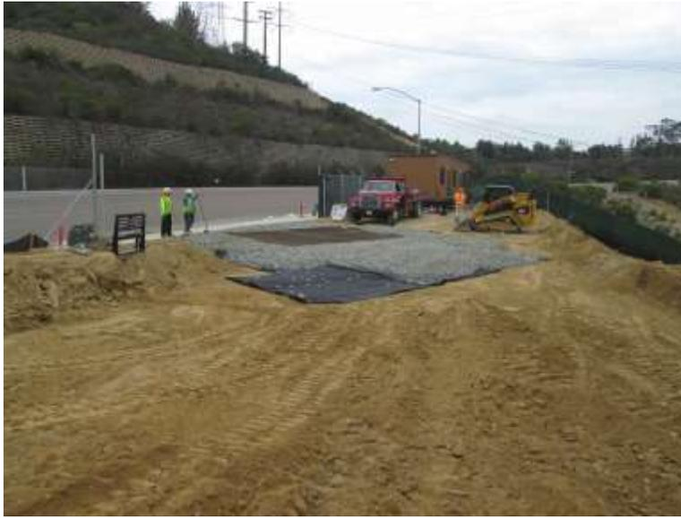
**Photo 3:** Trac-out control measures have been installed at the construction site entrance in accordance with the SWPPP and MM-HYD-1. Trac-out controls consisted of rattle plates and a rock apron in order to minimize trac-out onto paved public roads.
