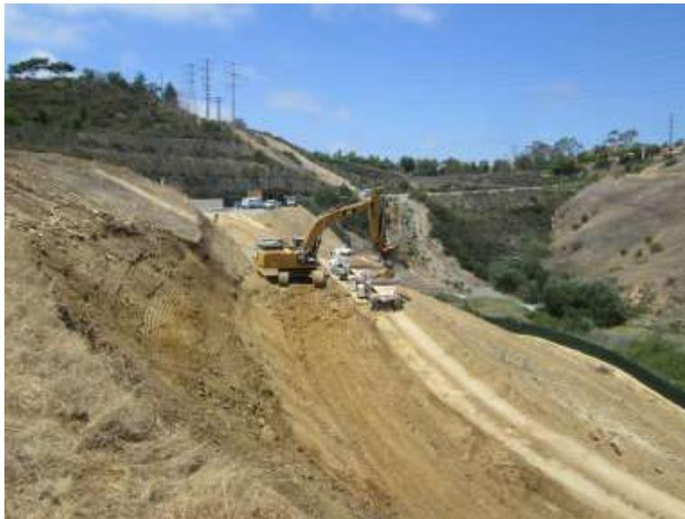
**Photo 2:** Soil being exported off site via the use of an excavator loading haul trucks.
