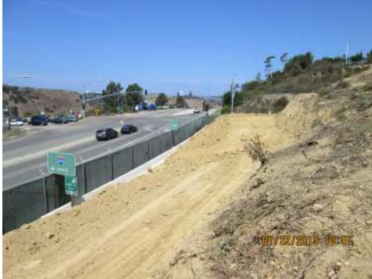
**Photo 1:** An access road has been established along the perimeter of the project site to provide access for haul trucks exporting soil off site.
