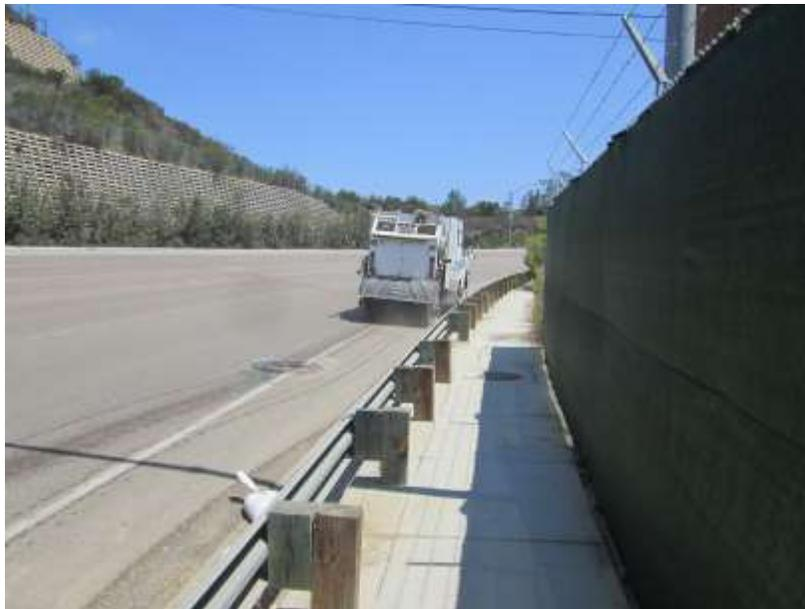
**Photo 4:** A street sweeper cleans paved roadway surfaces adjacent to the project site to remove trac-out in accordance with the SWPPP and MM-HYD-1.
