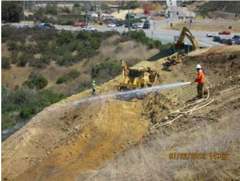
**Photo 3:** Water is utilized in areas of active construction to minimize fugitive dust emissions.
