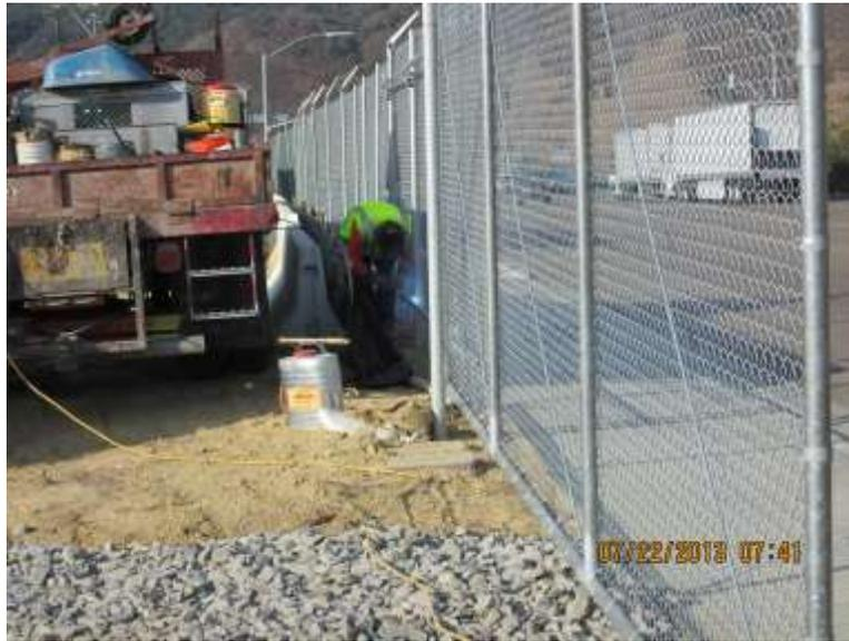
**Photo 5:** Fire suppression equipment consisting of a fire extinguisher and backpack pump was on site during welding activities in accordance with Mitigation Measure HAZ-2.
