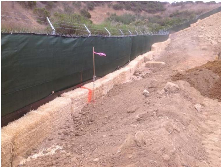
**Photo 4:** BMP's consisting of hay bales and silt fence installed along the downslope perimeter of the project site in accordance with the Stormwater Pollution Prevention Plan (SWPPP) and MM-HYD-1.
