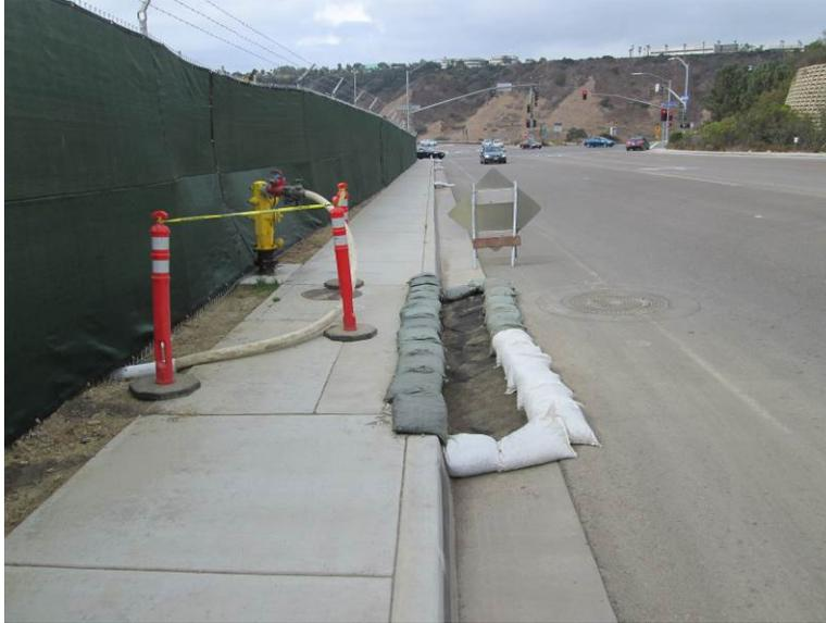
**Photo 3:** Check dams and inlet protection measures consisting of filter fabric were observed being maintained along Mira Sorrento Place in accordance with APM-HYD-1.
