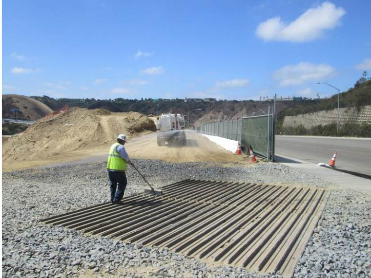
**Photo 4:** Trac-out measures consisting of a rattle plate and rock apron are being maintained at the construction site entrance in accordance with APM-HYD-1.
