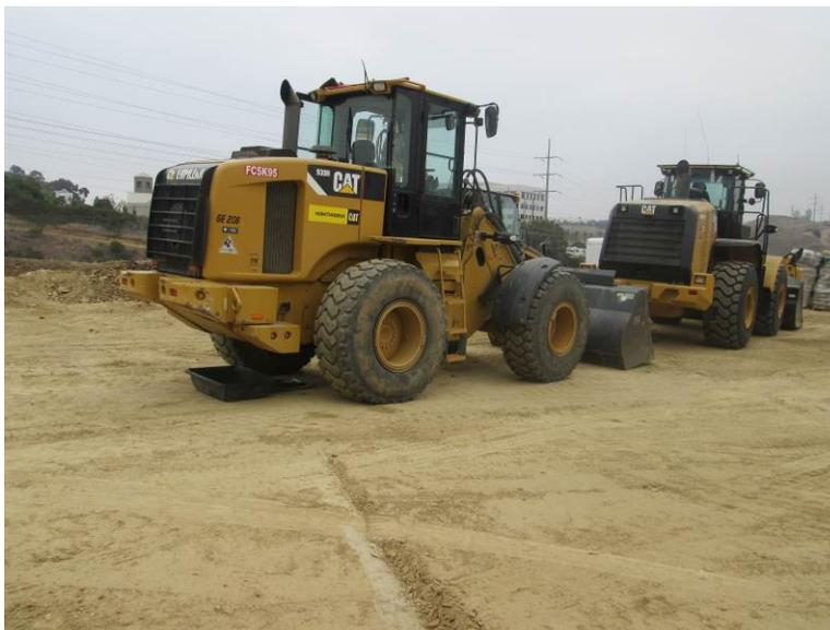
**Photo 2:** In accordance with APM-HYD-1, drip pans were observed beneath construction equipment to minimize the potential for oils and lubricants from the construction equipment to be discharged into soils.
