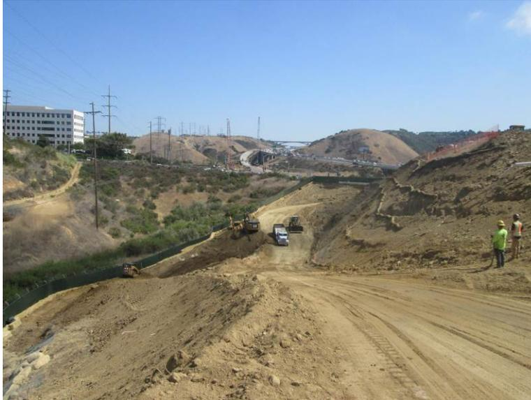
**Photo 1:** Construction activities associated with exporting soil offsite continued during this reporting period. Excavators were observed loading haul trucks to export soil offsite.
