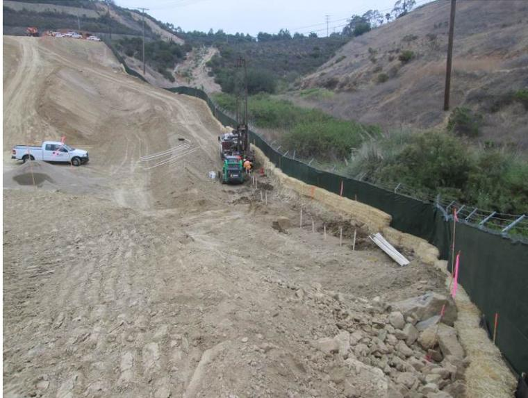
**Photo 1:** A series of groundwater wells were drilled along the eastern limits of the project site that will be utilized for groundwater extraction.
