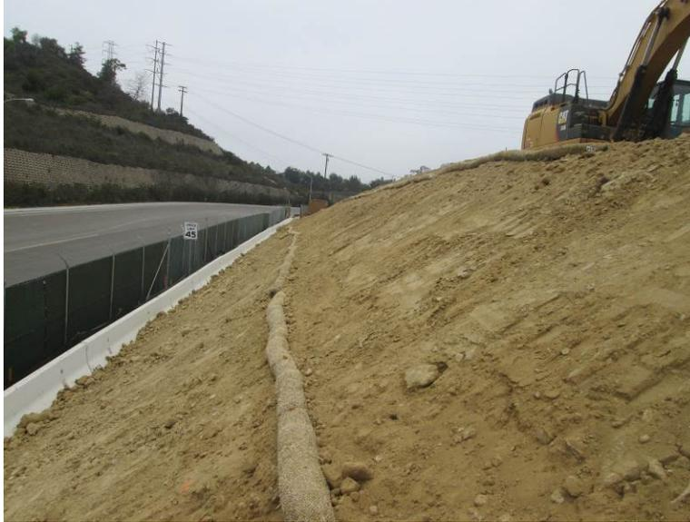
**Photo 3:** In accordance with APM-HYD-1, storm water control BMPs were observed along the site perimeter to minimize erosion and silt laden runoff.
