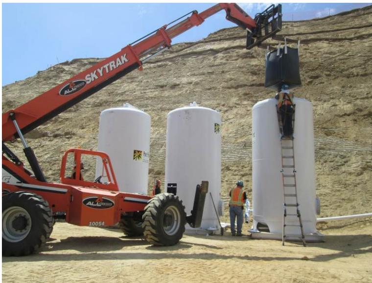
**Photo 2:** Filter tanks were observed being placed onsite to filter groundwater being extracted prior to any discharges offsite.
