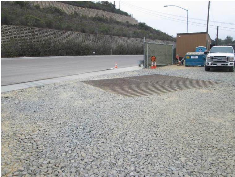
**Photo 6:** In accordance with APM-HYD-1, anti-dirt tracking control BMPs including a rock apron and rumble plates, were observed at the site ingress/egress point to prevent dirt from being tracked onto Mira Sorrento Place.
