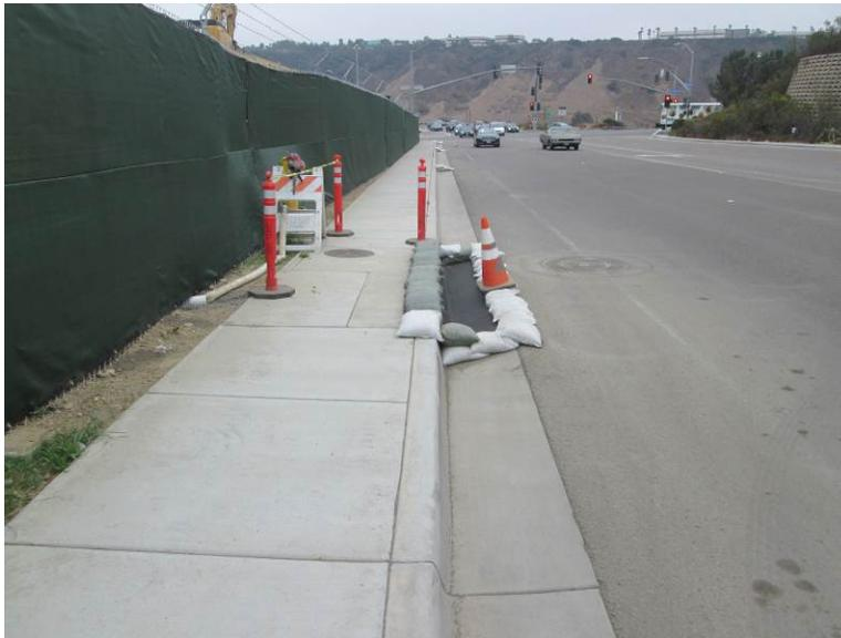
**Photo 4:** In accordance with APM-HYD-1, inlet protection BMPs designed to avoid or minimize silt from entering waterways, including filter fabric and gravel bags, were observed at two inlets along Mira Sorrento Place.
