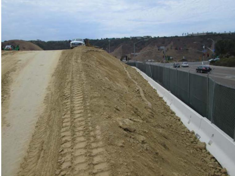
**Photo 5:** In accordance with APM-HYD-1, storm water control BMPs were observed along the site perimeter to minimize erosion and silt laden runoff.
