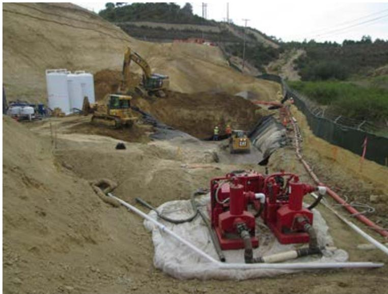
**Photo 4:** In accordance with APM-HYD-1, secondary containment was placed under staged construction equipment to prevent potential leaks from being discharged into the soil.
