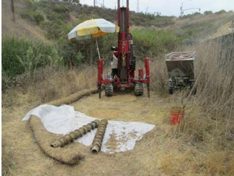
**Photo 3:** In accordance with APM-HYD-1, a straw wattle was placed between the wetland habitat and the groundwater monitoring wells for sediment control while decommissioning activities took place.
