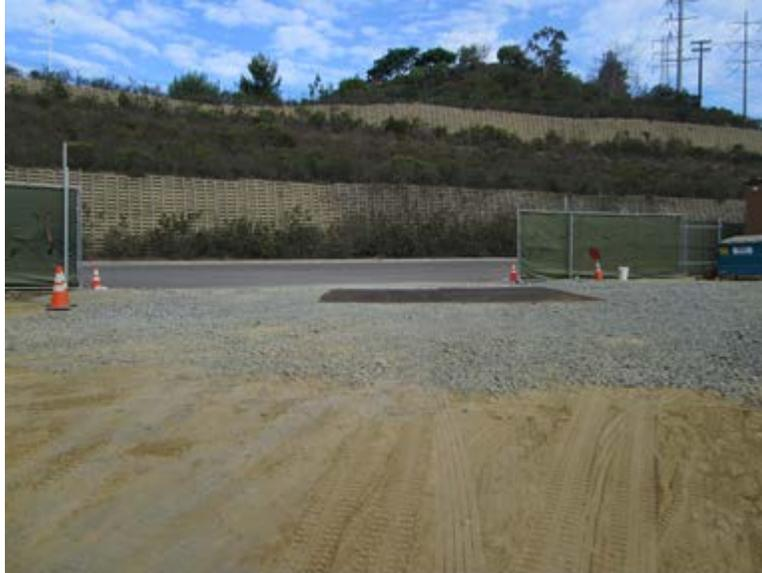
**Photo 6:** In accordance with APM-HYD-1, drip pans were used under construction equipment to prevent potential leaks from being discharged into the soil.
