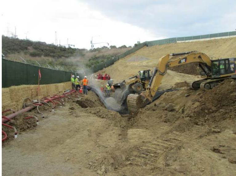
**Photo 1:** Dewatering continued along the eastern perimeter of the construction site, as soil saturated with groundwater was excavated and replaced with gravel fill in preparation for wall construction.
