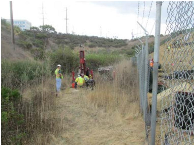
**Photo 2:** Decommissioning of two groundwater monitoring wells outside the project limits and adjacent to the wetland ESA.
