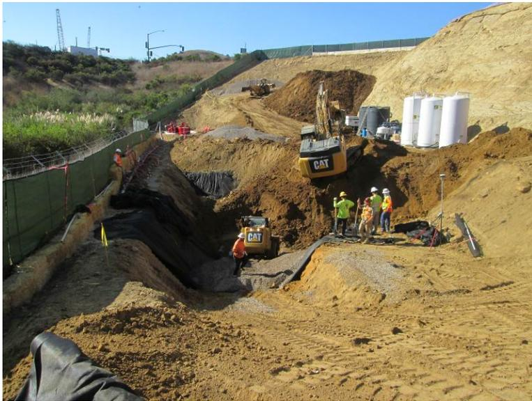
**Photo 2:** Soil saturated with groundwater, adjacent to the groundwater dewatering wells, was excavated and replaced with gravel fill in preparation for wall construction.
