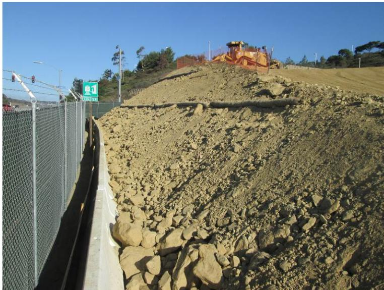
**Photo 4:** In accordance with APM-HYD-1, storm water control BMPs were observed along the site perimeter and on open cut slopes to prevent silt laden water from entering waterways.
