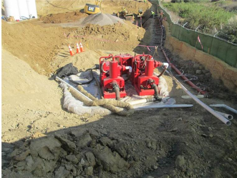
**Photo 3:** In accordance with APM-HYD-1, secondary containment is placed beneath staged construction equipment to prevent potential leaks from being discharged into the soil.
