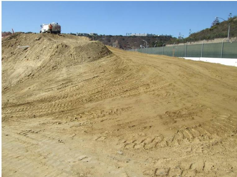
**Photo 6:** In accordance with APM-HYD-1, water was applied to the work area and to access roads to prevent wind erosion and dust creation.
