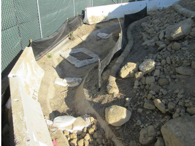
**Photo 5:** In accordance with APM-HYD-1, inlet protection BMPs were utilized at all applicable storm drains to prevent sediment laden water from entering waterways.
