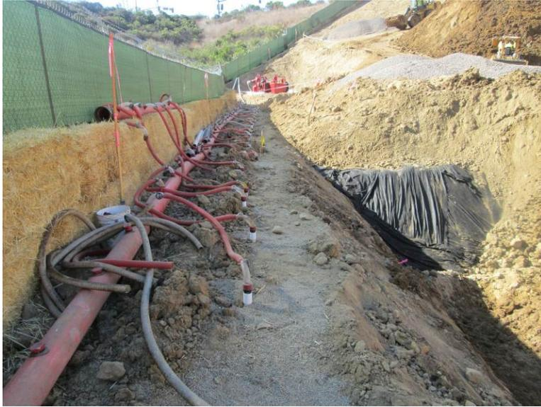
**Photo 1:** Groundwater wells constructed along the eastern limits of the project site.
