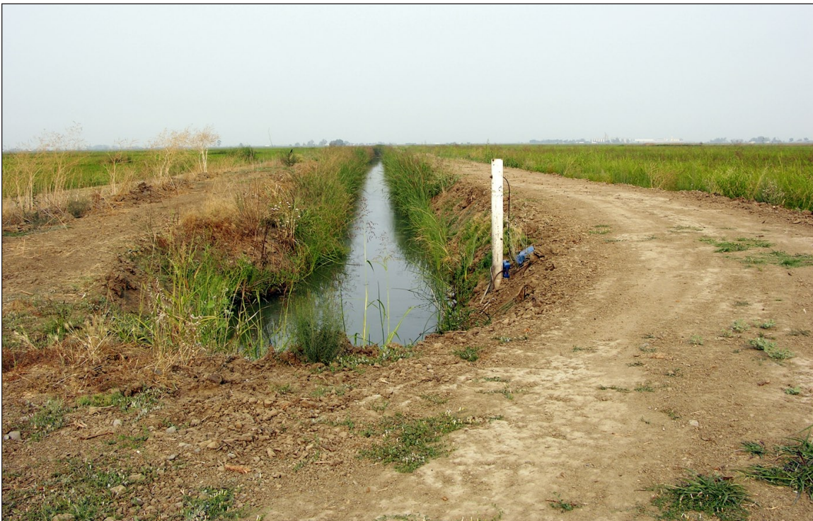
Photo 6. Typical irrigation ditch that occurs throughout rice fields in the project area. The pipeline will be installed across most of these small irrigation ditches and canals using an open-cut trench method.
