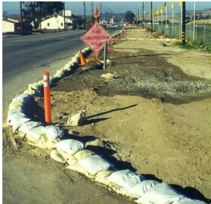
Sand bags used as perimeter control.
