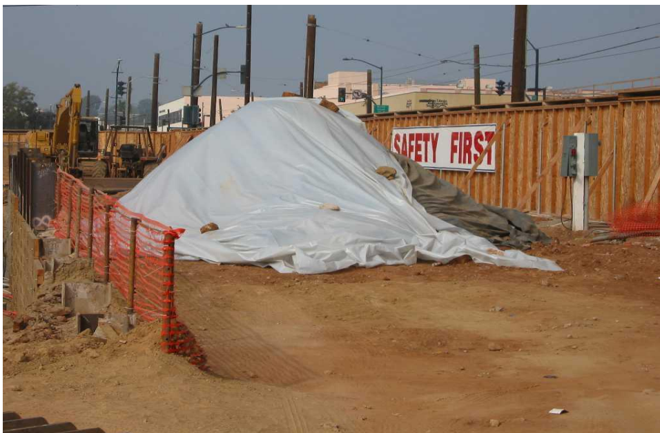
Stockpile covered with plastic and secured with large rocks.
