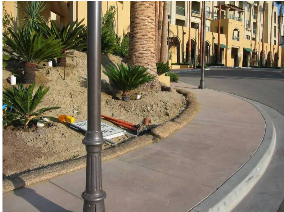
Fiber rolls as perimeter control.
