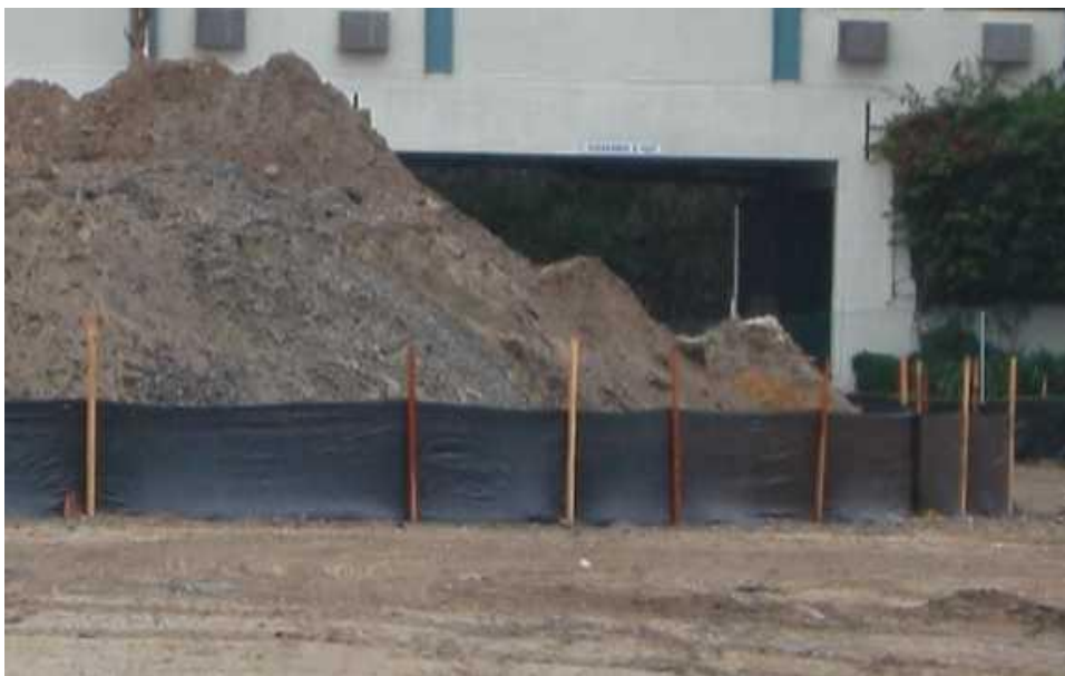
Silt fence used for stockpile perimeter control.
