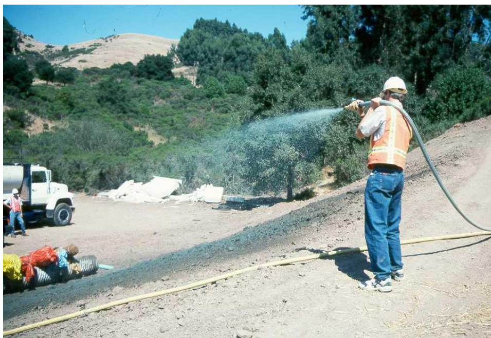
Applying hydroseed.
