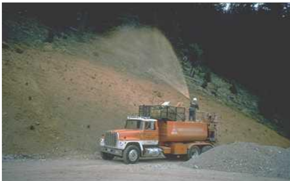
Applying hydraulic mulch.
