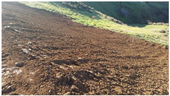
Photo 3: Provide cover for inactive slope and place fiber rolls every 10 ft. and trench in fiber rolls at the Natural Substation, February 9, 2015
