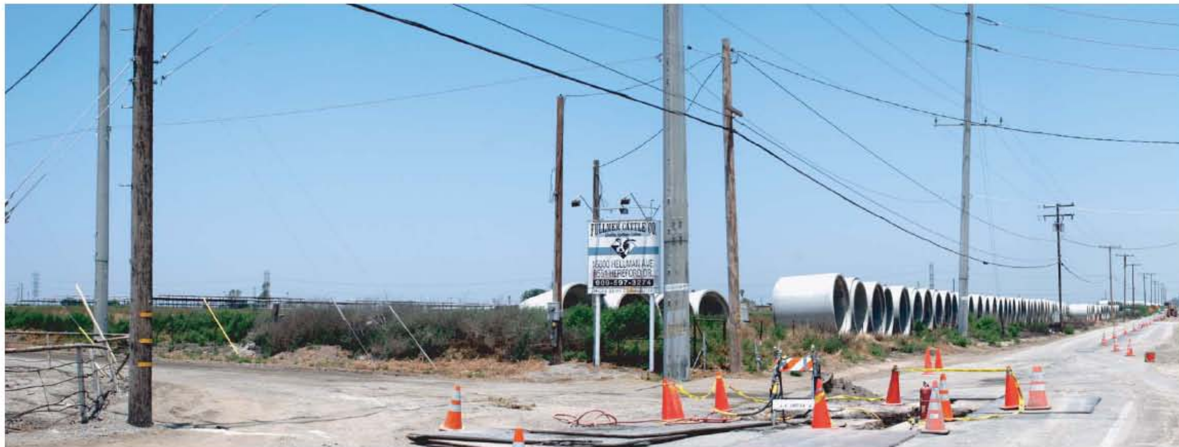
Existing Condition: Viewing north along Hellman Avenue
