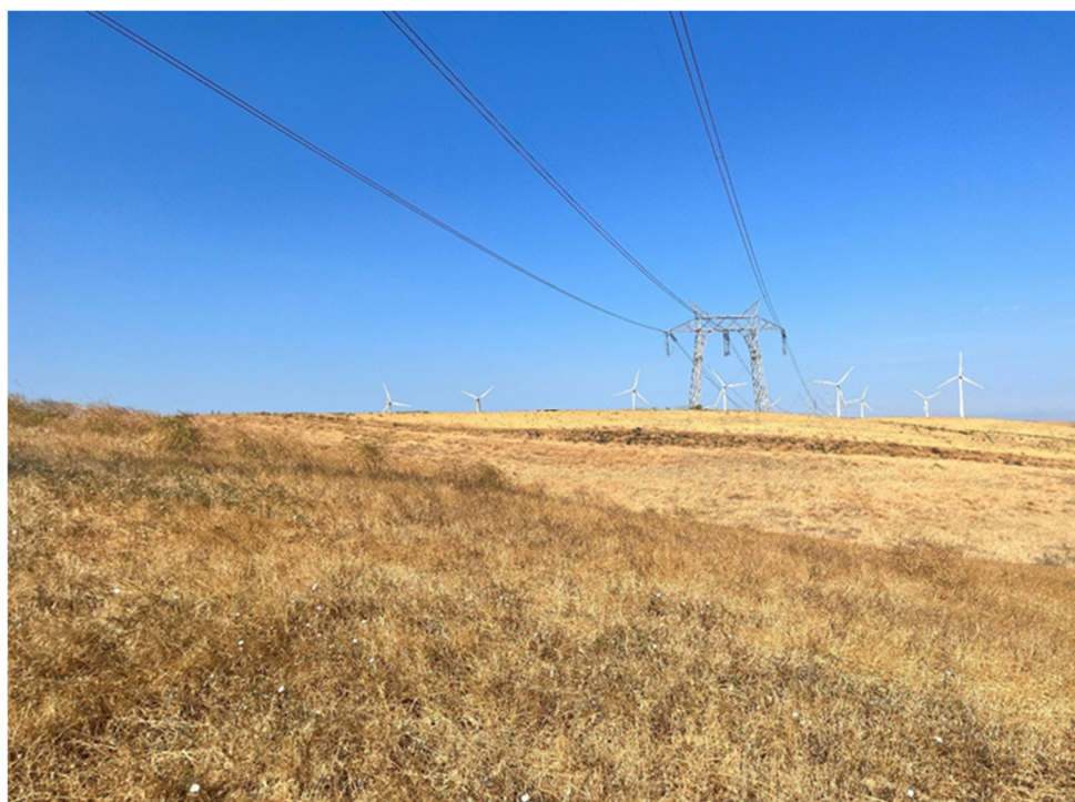
Figure 6-1 . Proposed Project overview, facing southwest.
