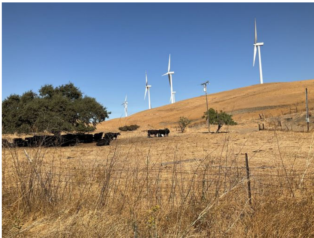
Figure 7-13. Site overview, facing north.
