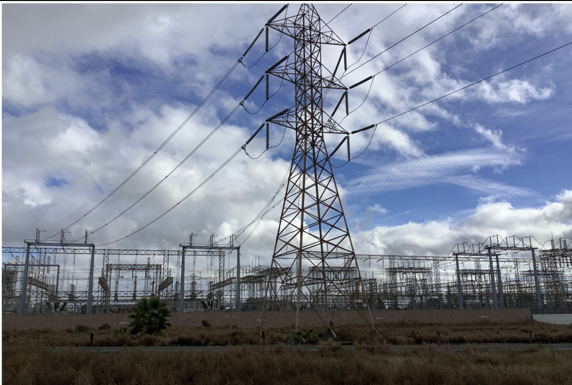
Figure 7-16. Overview of P-07-002956. View east.
