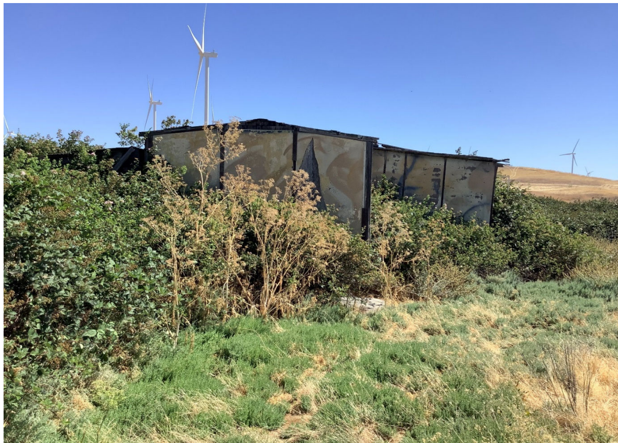
Figure 7-22. Site overview, facing northeast.
