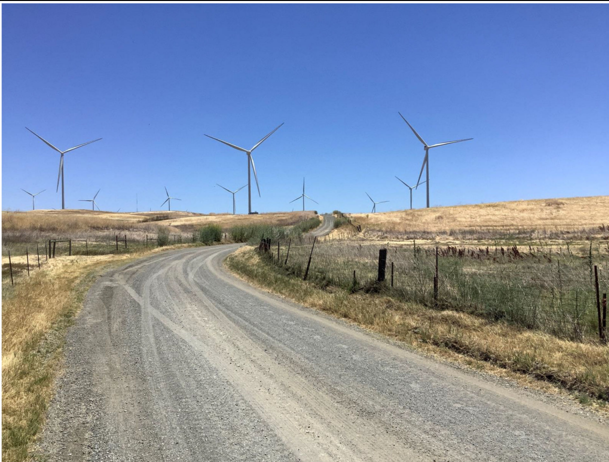
Figure 7-24. Overview of Stratton Lane, Segment 1, view east.
