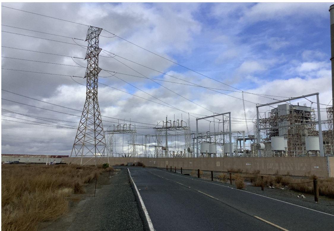
Figure 7-15. Overview of P-07-002956. View north.
