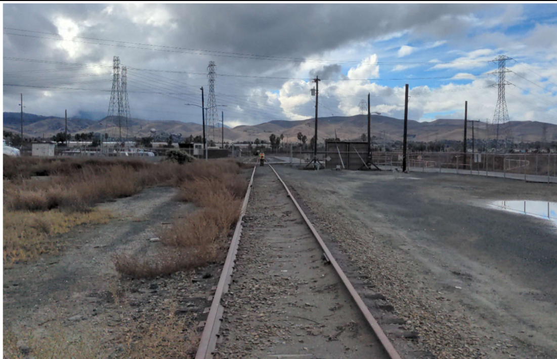
Figure 7-21. Overview of the Burlington Northern Santa Fe Railway line. View north-southeast.
