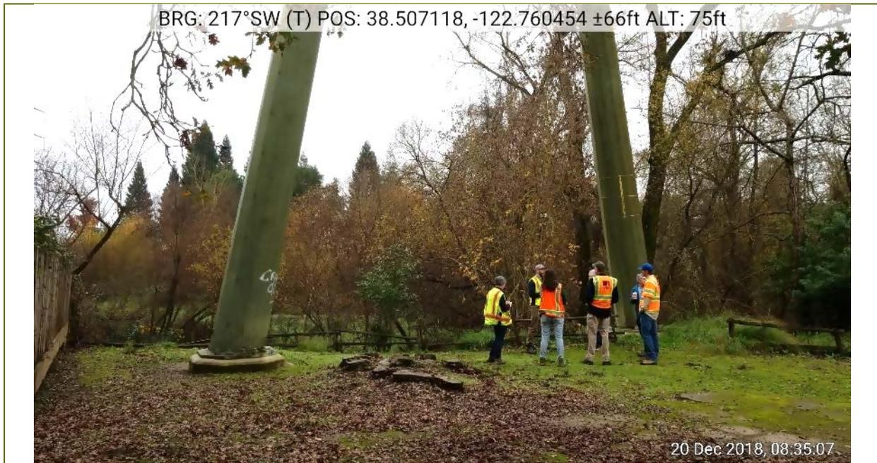
Pole 13 (double shaft-structure) is positioned just above the bank of Mark West Creek. The two existing poles would be replaced with two separated poles positioned farther away from the creek bank (see Figure 1). Construction would occur on the flat area in view and not within the creek channel or riparian vegetation beyond the existing poles.
