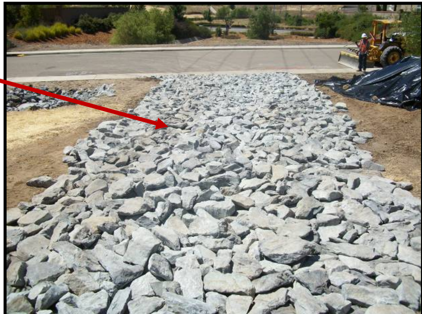
Traditional rocked construction entrance/exit.
