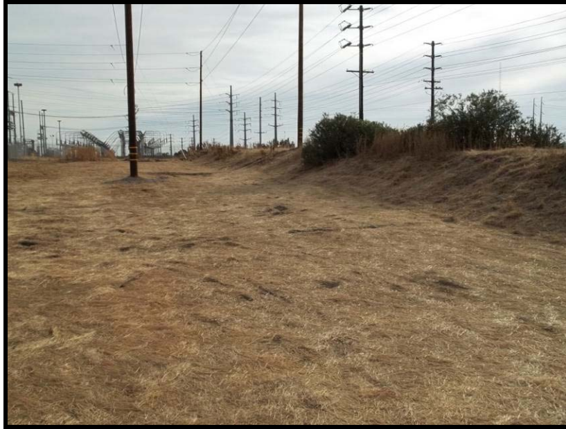
Straw mulch protecting a disturbed area.
