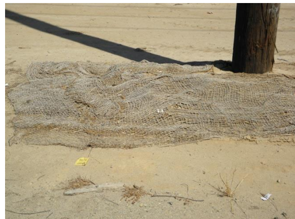
Stabilized disturbed soil
