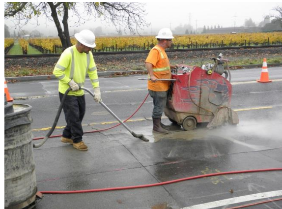
Sawcutting in preparation of Excavation
