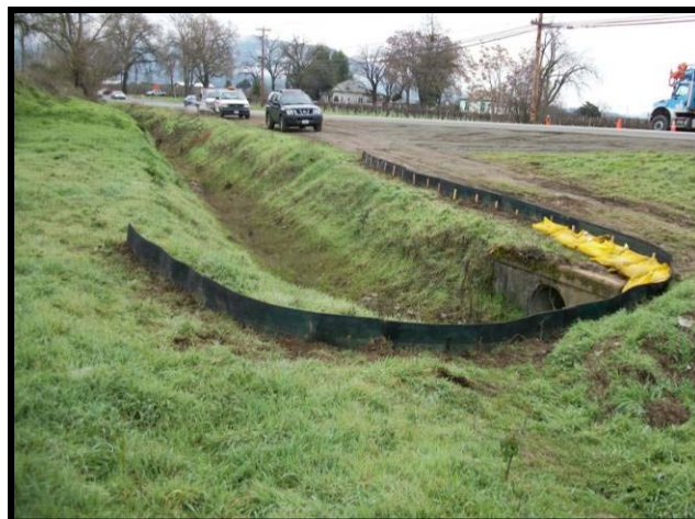
Silt fence reinforced with gravel bags.
