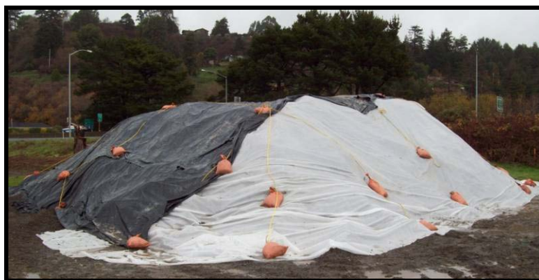
Proper securing of plastic sheeting.
