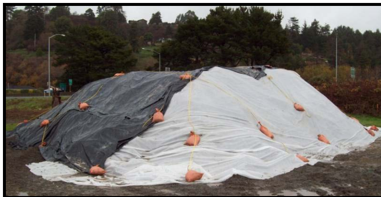
Proper securing of plastic sheeting.
