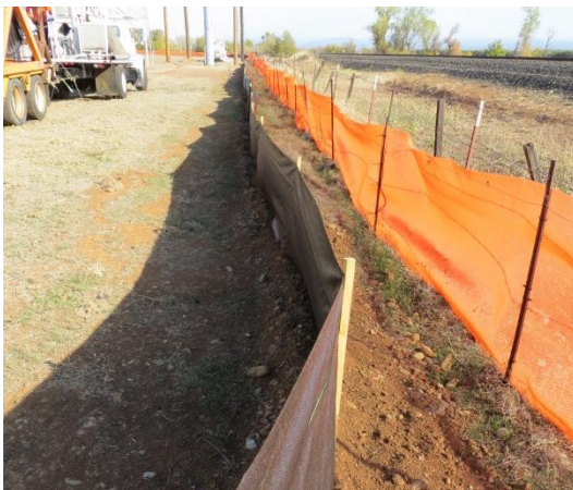
Perimeter control and fencing in place
