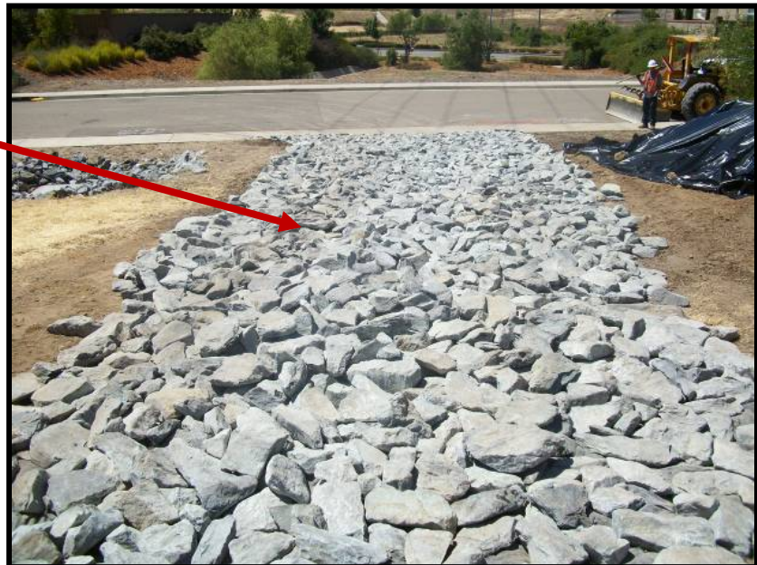
Traditional rocked construction entrance/exit.
