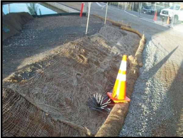
Fiber roll at foot of slope and protecting channel prior to pole replacement.
