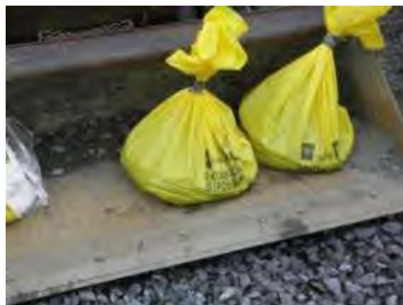
Contaminated soil properly prepared for disposal
