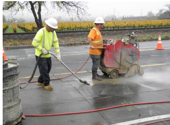
Proper sawcutting procedure
