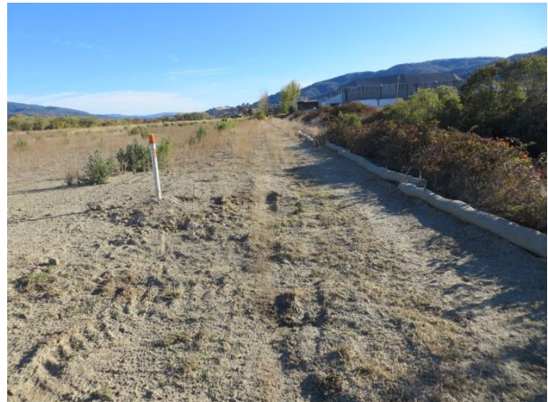
Perimeter control in place
