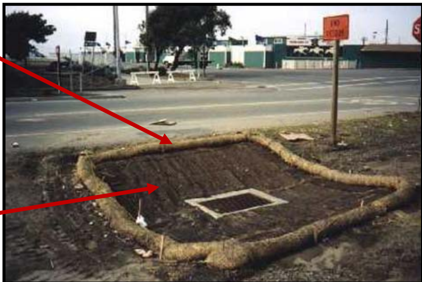
Straw fiber rolls combined with geotextile fabric for drain inlet protection.
