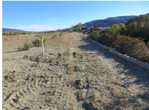
Perimeter control in place
