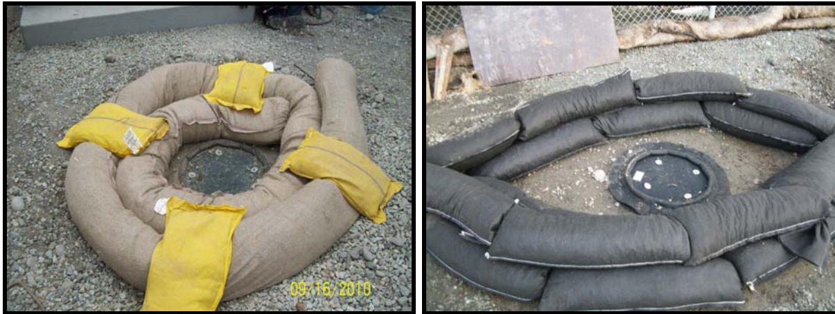
Additional methods of inlet protection using fiber rolls and gravel bags.
