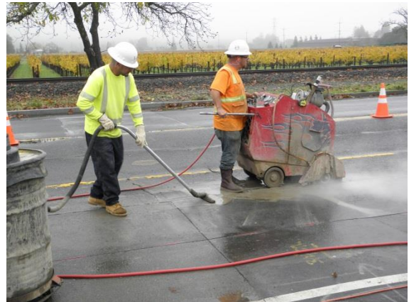
Sawcutting in preparation of Excavation
