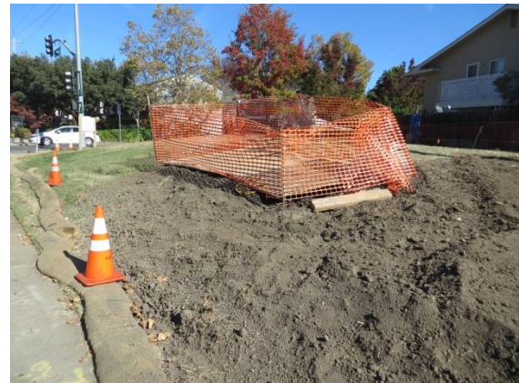
Excavation covered for safety at end of day
