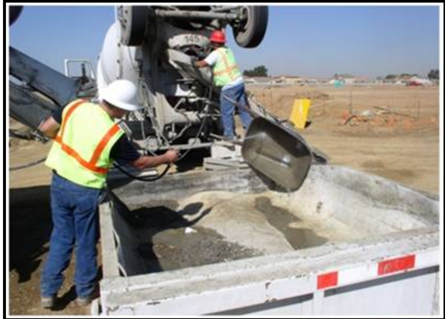
Self contained concrete washout.
