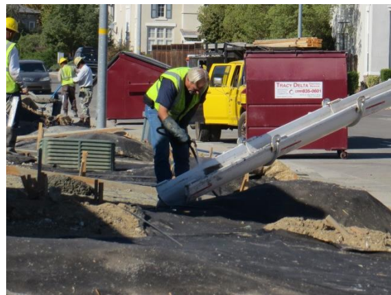
Concrete placement
