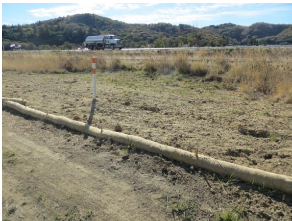
Stabilized disturbed soil with perimeter treatment
