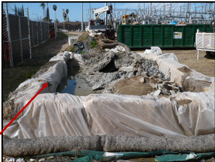
Lined concrete washout.
