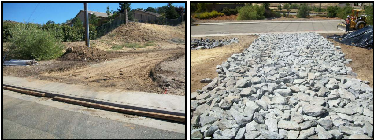
Construction entrance/exit before and after installation.
