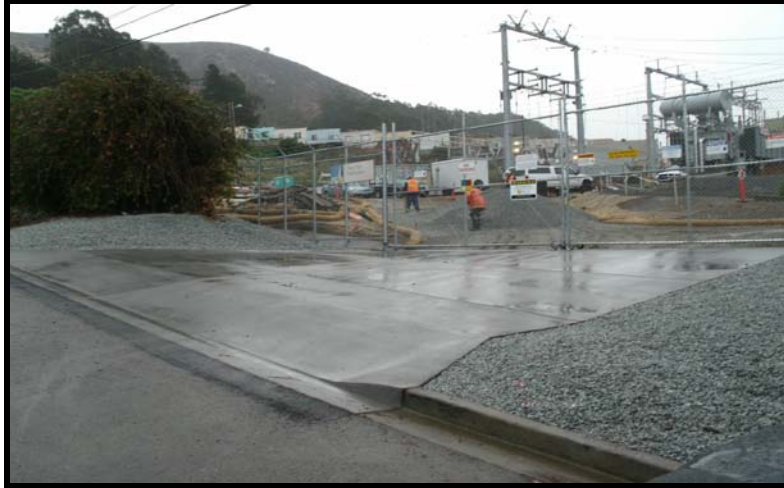
Clean and well maintained construction entrance/exit.
