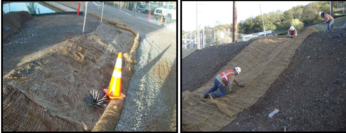
Jute mat used to protect soil on slope and embankment.
