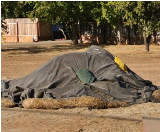
Figure 5. Contaminated stockpile under cover
