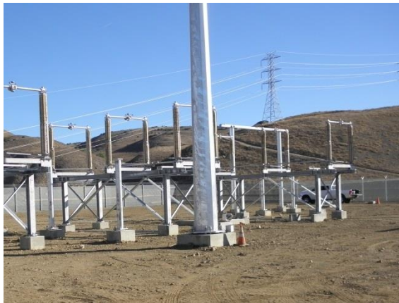
Pole with concrete footing
