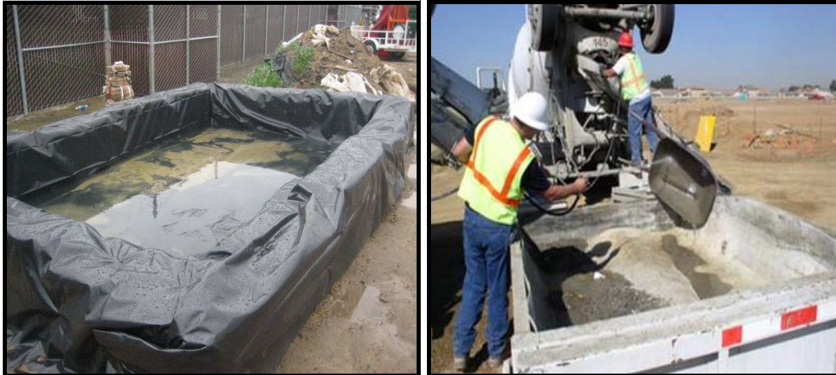
Two alternatives for containing concrete washout water.
