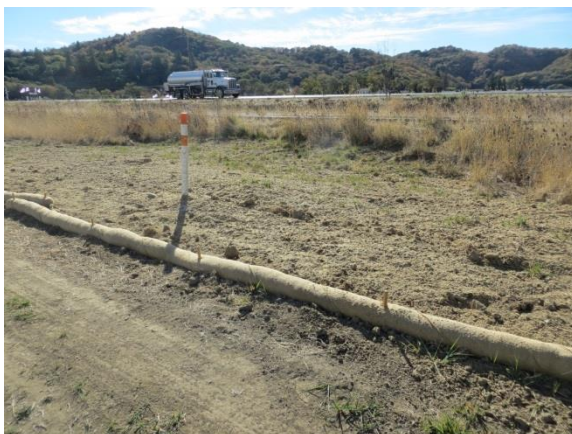
Stabilized disturbed soil with perimeter treatment
