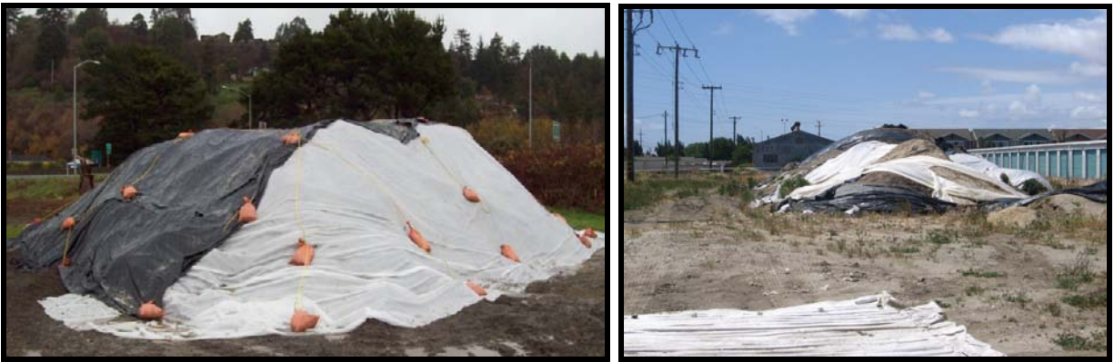
Plastic sheeting over stockpiles properly and improperly secured.
