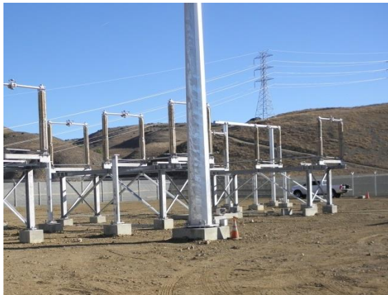
Pole with concrete footing
