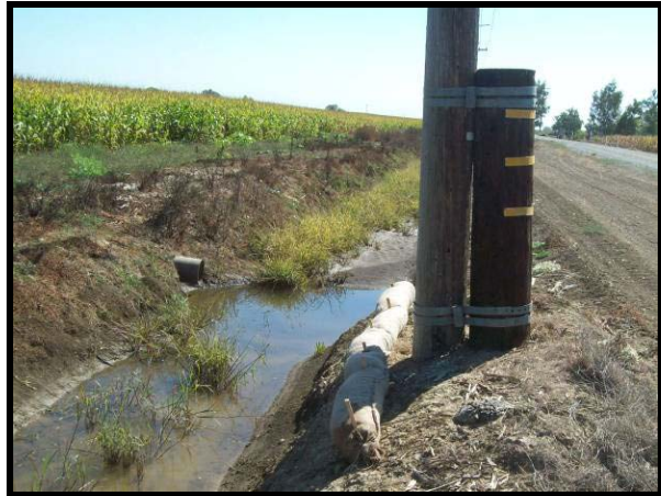
Fiber roll at foot of slope and protecting channel prior to pole replacement.
