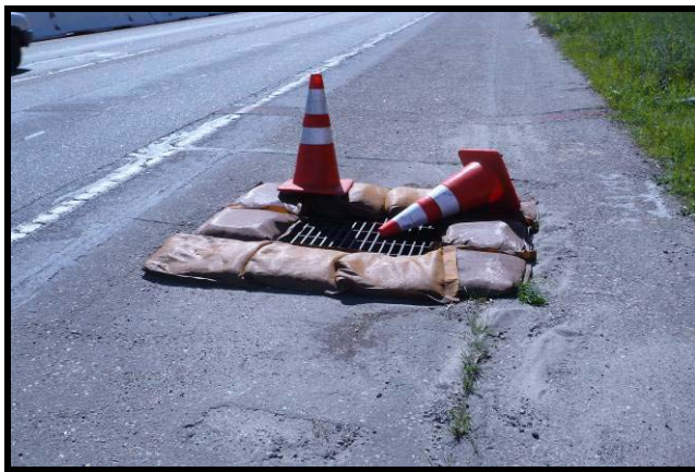
Appropriate inlet protection.
