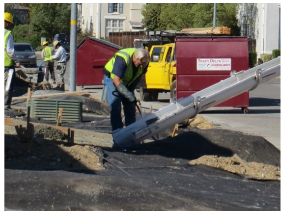
Concrete placement
