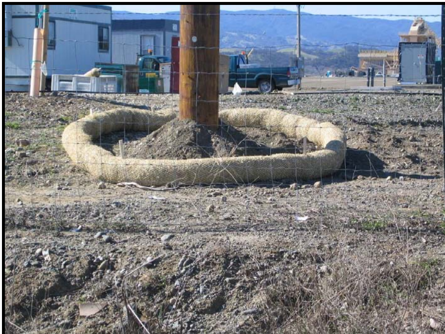
Fiber roll protecting a pole replacement site
