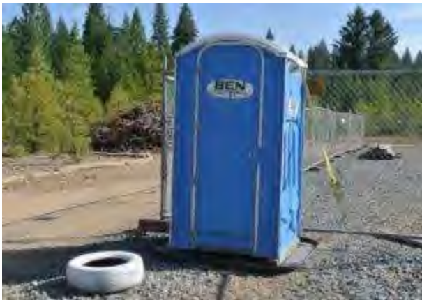
Properly placed on tray and tied down
