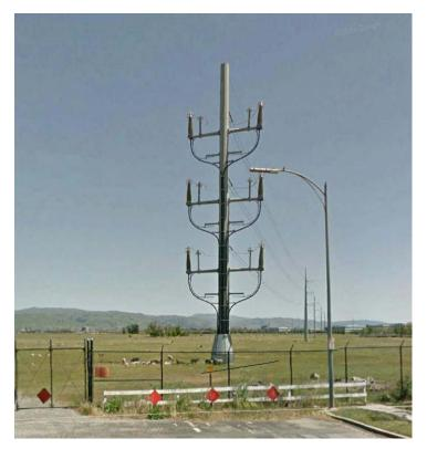
Figure 9- Silicon Valley Power 230-kV Riser
