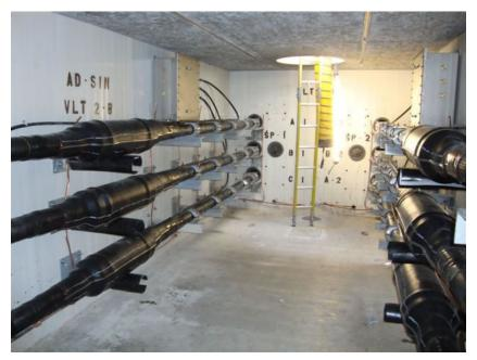
Figure 13 - Typical Cable Splice Vault
