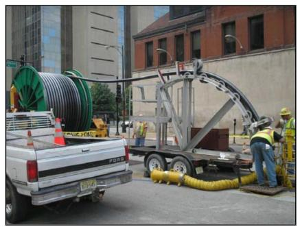
Figure 12 – Cable Pulling Arrangement
