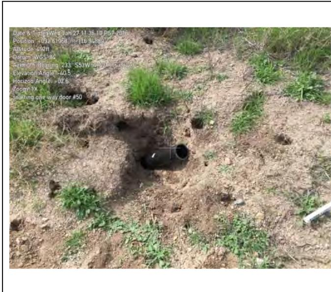
Photo 1. Insertion of 4 inch pipe prior to installation of one way door.
