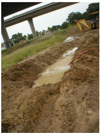
**Figure 6** – Dewatering ditch created to contain groundwater from the Pole 2/15 foundation hole, May 17, 2005.
