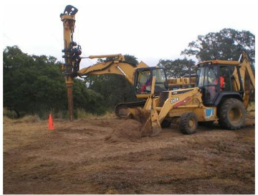
**Figure 1** – Pole 20 area, June 8, 2005. Note the backhoe clearing auger spoils.
