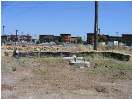
**Figure 1** – Pole 22, July 5, 2005. Note the hay bales and sediment fence located beyond the pole location which protects a sensitive vernal pool area.
