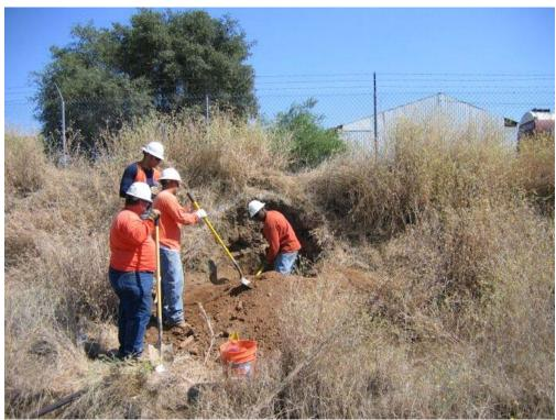
**Figure 1** – Crews pot-holing at pole site #5 adjacent to the railroad, July 27, 2005.
