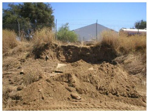
**Figure 2** – Crews covered the 15-foot deep augured foundation hole at Pole 5 adjacent to the railroad, August 6, 2005.
