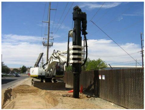
**Figure 1** – Crews auguring the foundation hole at the Pole 1 site, August 9, 2005.
