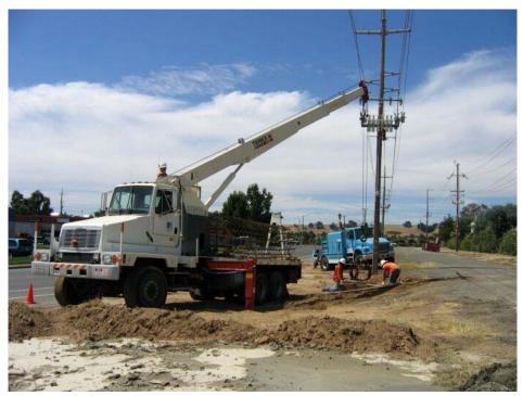
**Figure 2** – Crews installing the foundation cage at the Pole 2 site, August 9, 2005. Note the bermed area in the foreground into which groundwater was pumped.
