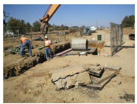
**Figure 1** – Vault installation with extending trench line north of Farron Street, September 15, 2005.
