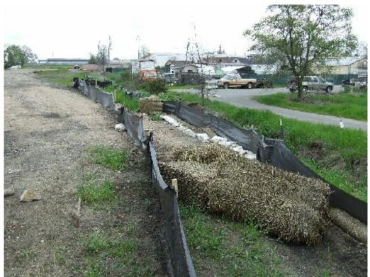
Figure 2 – Bank of Drainage #30 with newly installed erosion control features, March 30, 2006.
