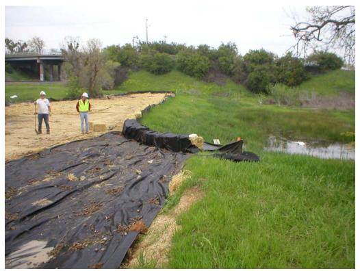
**Figure 1** – Erosion controls installed to filter the storm water runoff from the alignment into the adjacent wetland, April 7, 2006.
