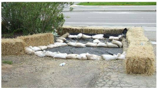
**Figure 1** – Erosion controls installed to filter the storm water runoff from the construction yard into the street and storm gutters, April 14, 2006.
