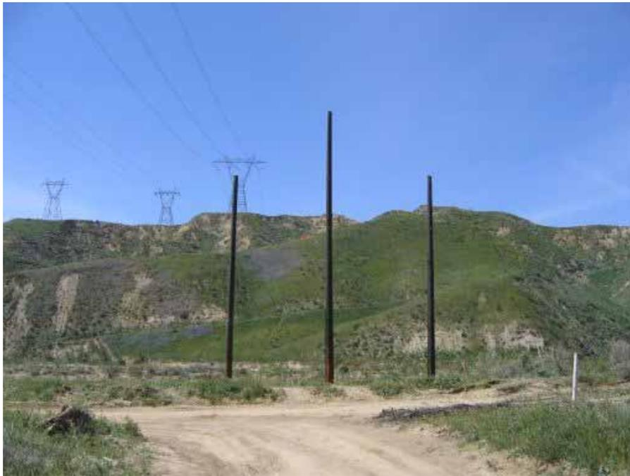
**Figure 3:** Three-pole Shoofly structure at Shoofly Location 13.
