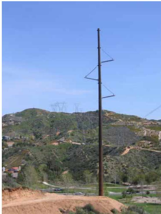
**Figure 2:** Typical one-pole Shoofly structure at Location 2.
