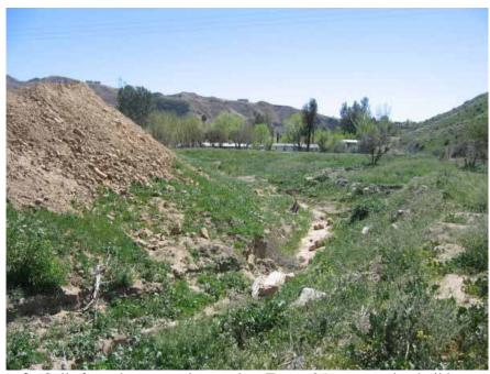
**Figure 2:** Soils from the excavation work at Tower 25 were used to build up earthen berms immediately adjacent to a dry drainage at the disposal site. Some material had slid into the channel, a Project Memorandum was issued by the CPUC EM for the non-compliance activity.
