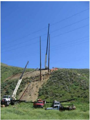
**Figure 1:** The installation of Shoofly poles at location 14 involved two cranes to move the poles up a steep slope.
